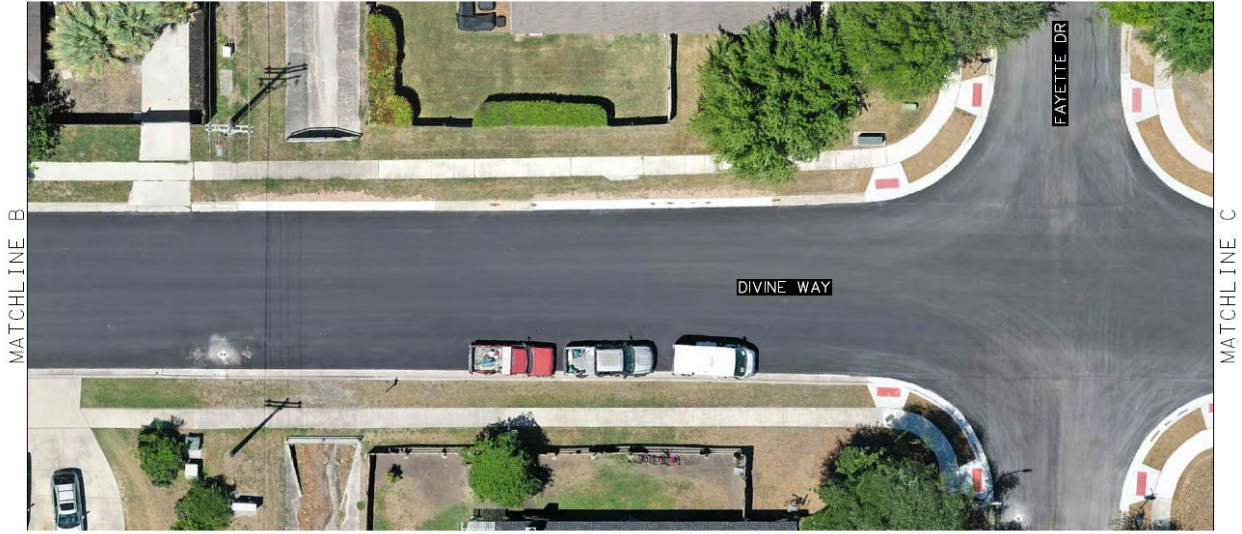
Figure 3 – Current, improved pavement and ADA ramps at the subject intersection following the 2023 Bond Citywide Street Improvements project.
