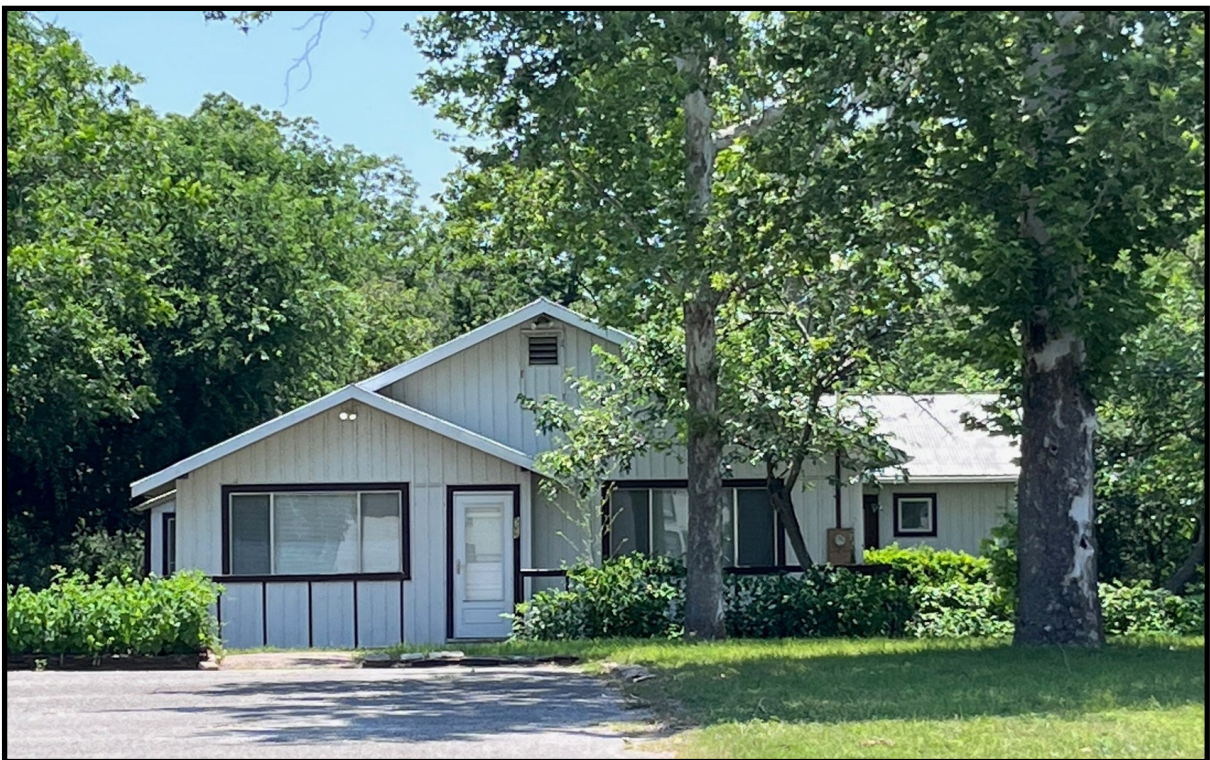
586 Granada Drive residence
