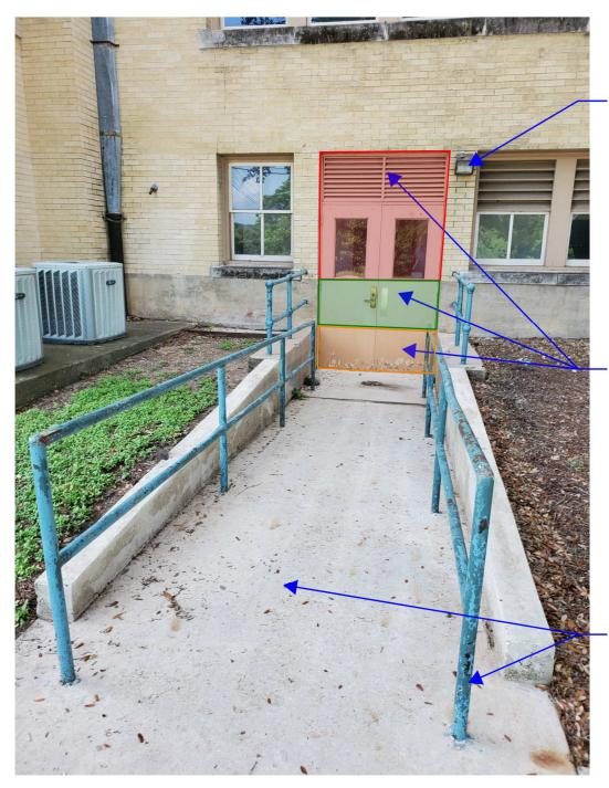
REMOVE LIGHT FIXTURE AND INFILL OPENING WITH MOTAR TO MATCH EXISTING GROUT COLOR
