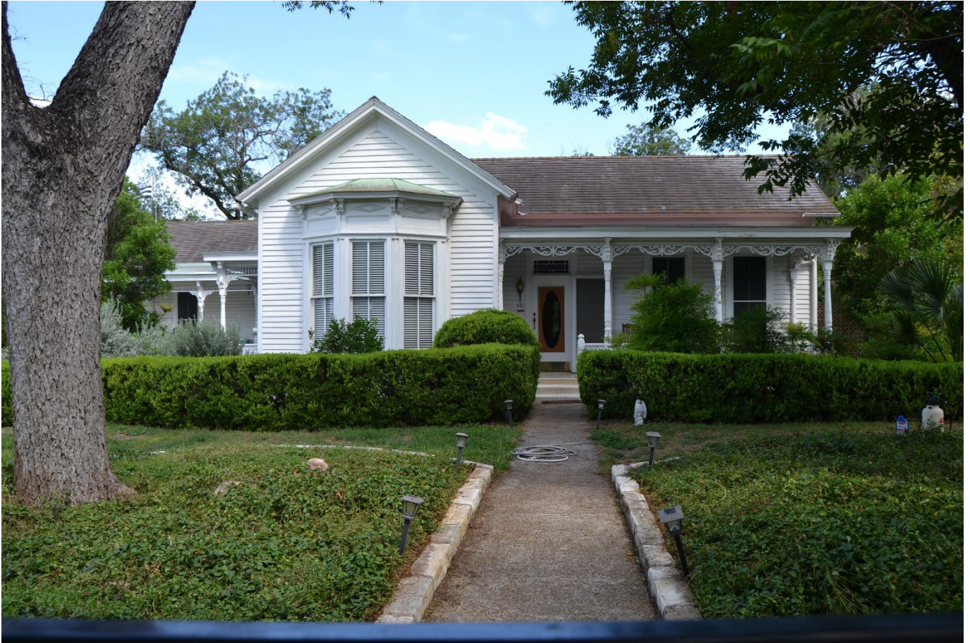
Photo 5. Front façade of the Liebscher House (Resource 1). Camera facing southeast.
