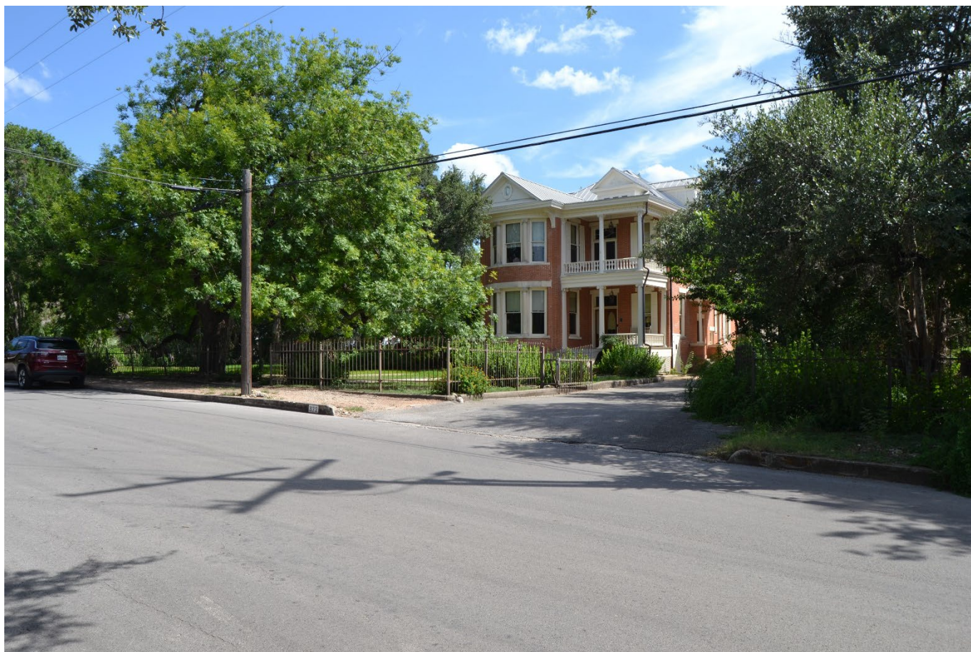
Photo 3. View of Dittlinger property and house (Resource 3) at 372 Magazine Avenue. Camera facing southeast.
