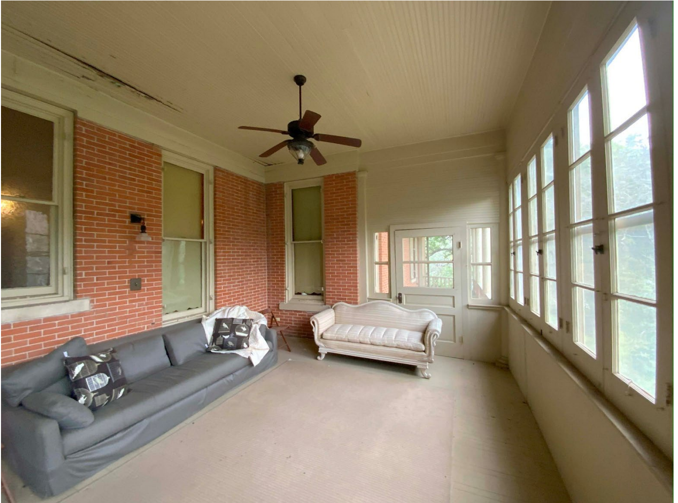
Photo 18. Rear portion of the second-story porch on the side southeast façade of the Dittlinger House (Resource 3). Camera facing northeast.
