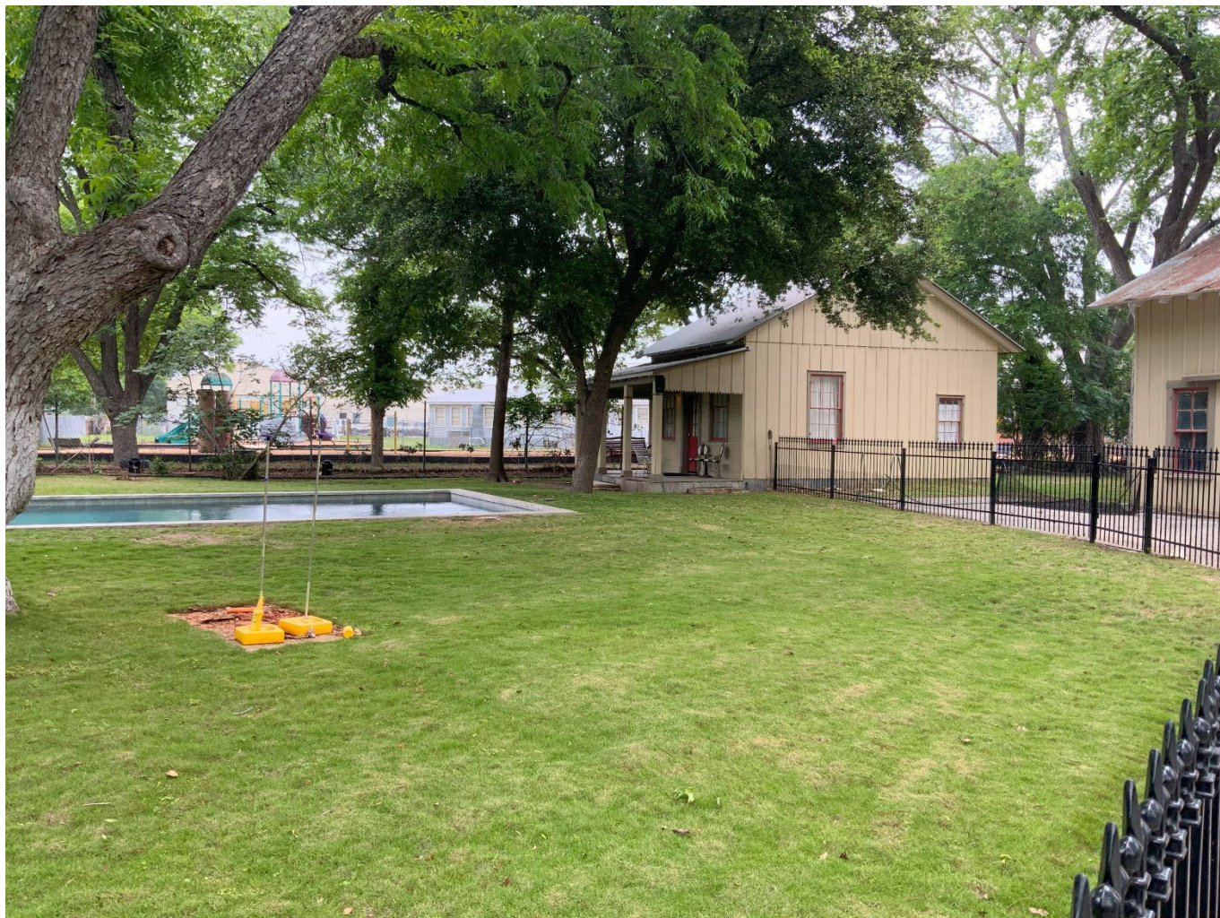
Photo 32. View of the side of the Professor's House backhouse (Resource 10) and pool (Resource 5) at 372 Magazine Avenue. Camera facing southeast.
