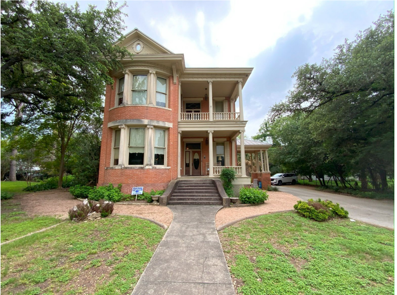
Photo 15. Front façade of the Dittlinger House (Resource 3) at 372 Magazine Avenue. Camera facing southwest.
