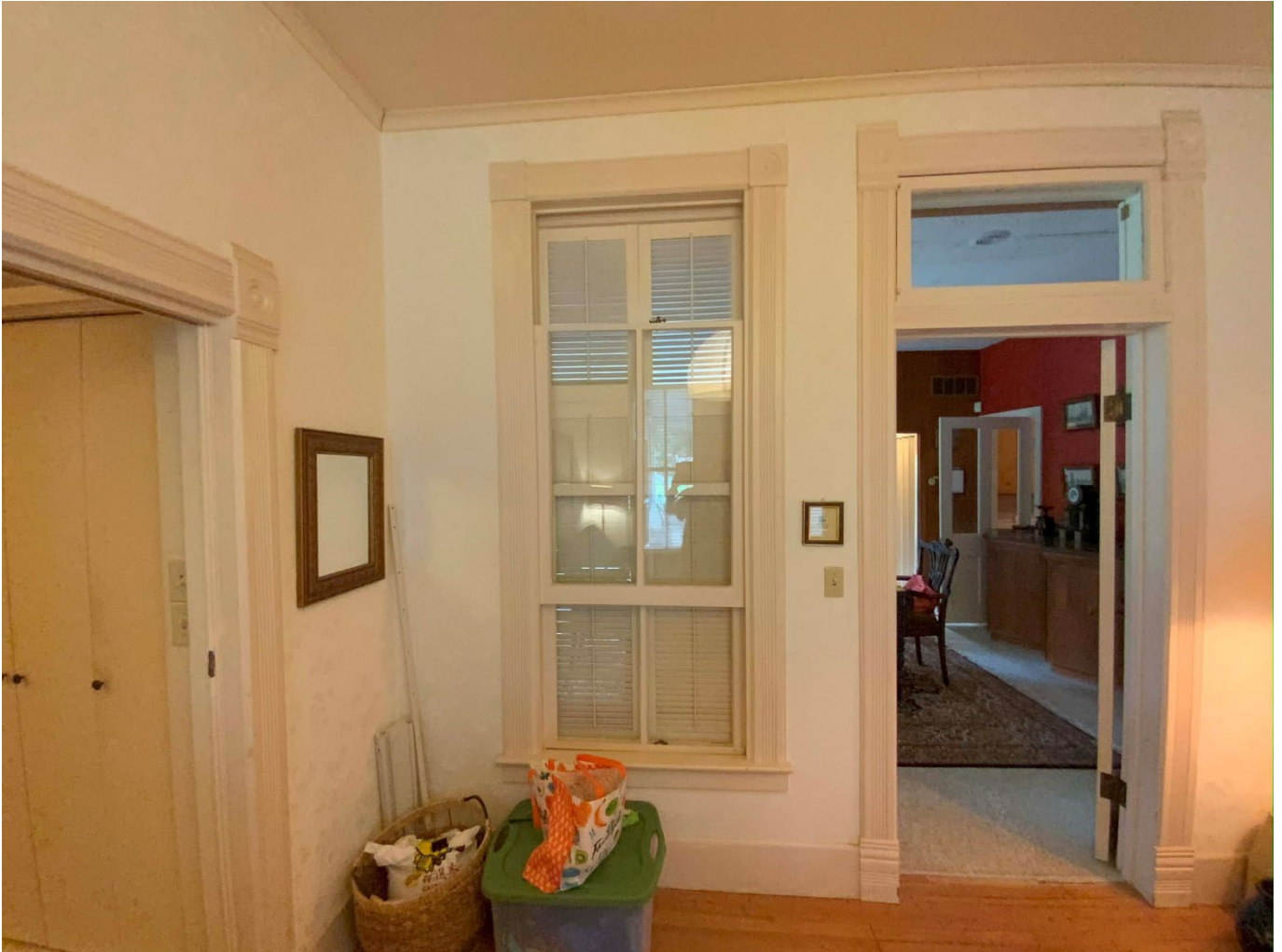
Photo 10. Interior view of the Liebscher House (Resource 1) showing an original rear wall with windows and door that became an interior wall with the 1963 addition. Camera facing northeast.
