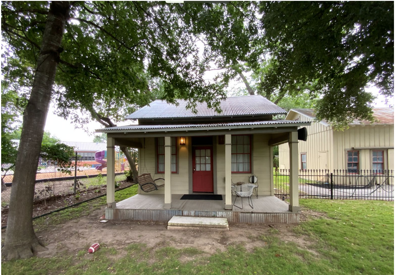
Photo 31. Front façade of the Professor's House backhouse (Resource 10) at 372 Magazine Avenue. Camera facing southwest.
