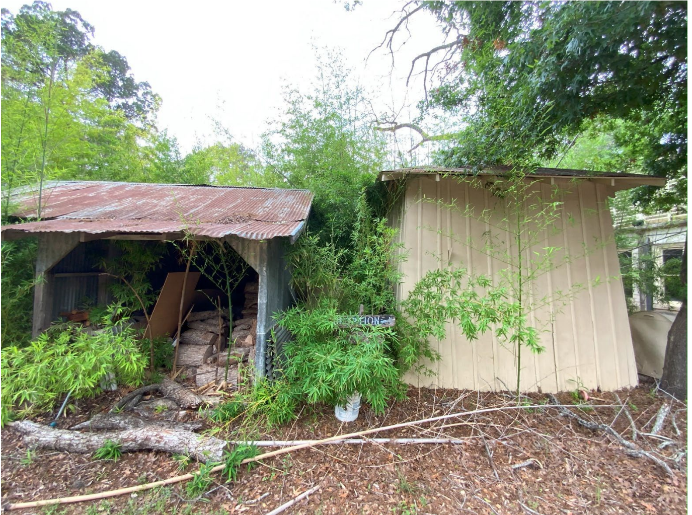
Photo 27. The shed (Resource 8) and pump shed (Resource 7) at 372 Magazine Avenue. Camera facing northwest.
