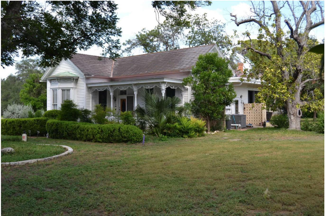
Photo 7. Oblique of the front of the Liebscher House (Resource 1). Camera facing northeast.
