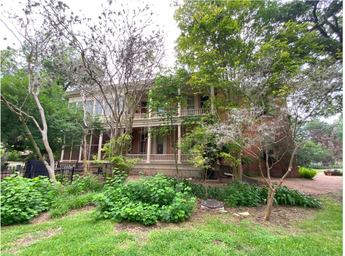
Photo 16. Side southeast façade of the Dittlinger House (Resource 3) showing the porches. Camera facing northwest.
