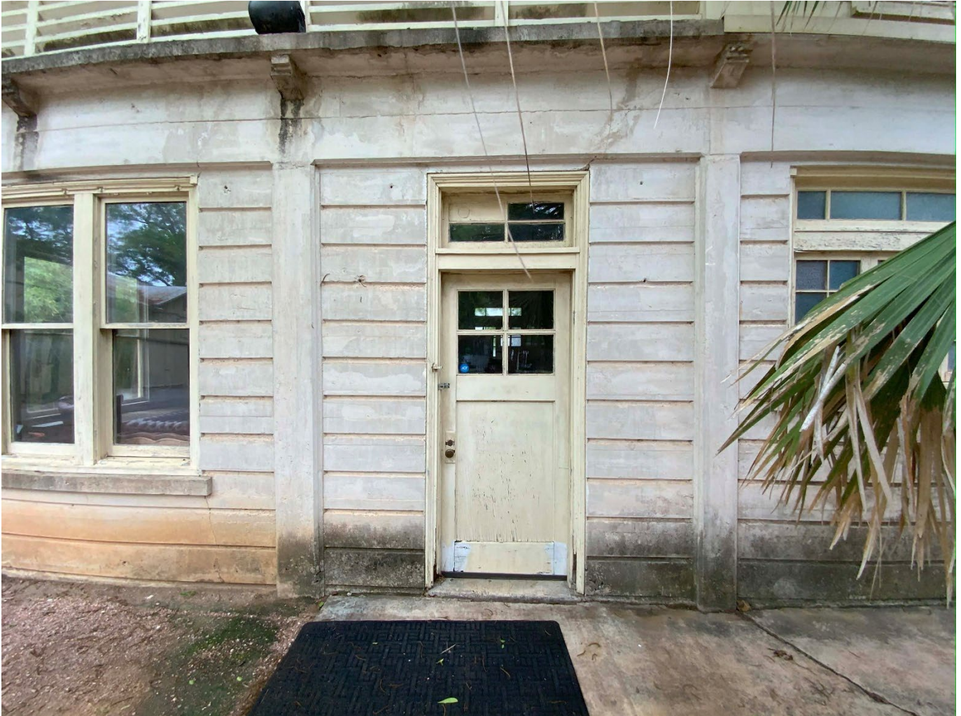
Photo 24. Detail of the concrete walls, pilasters, and brackets on the front façade of the wash house (Resource 4) at 372 Magazine Avenue. Camera facing northwest.
