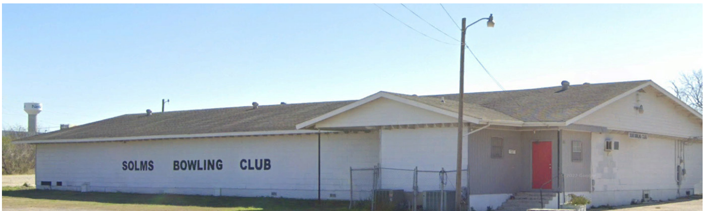
Solms Road Reconstruction Project - Solms Bowling Club
