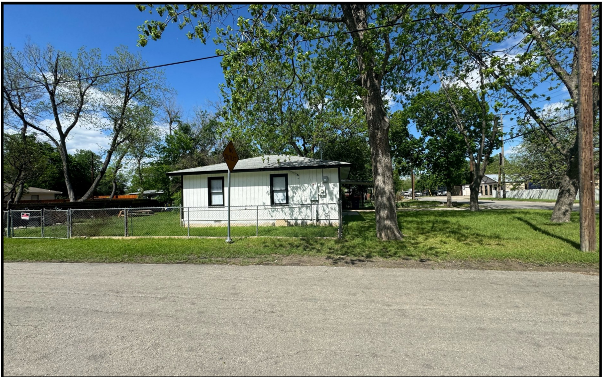
311 E Torrey St— N Central Ave Frontage
