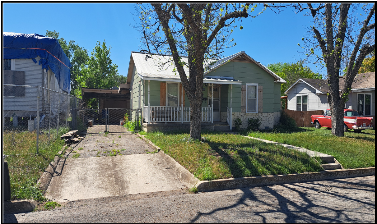
380 Kessler Street property frontage
