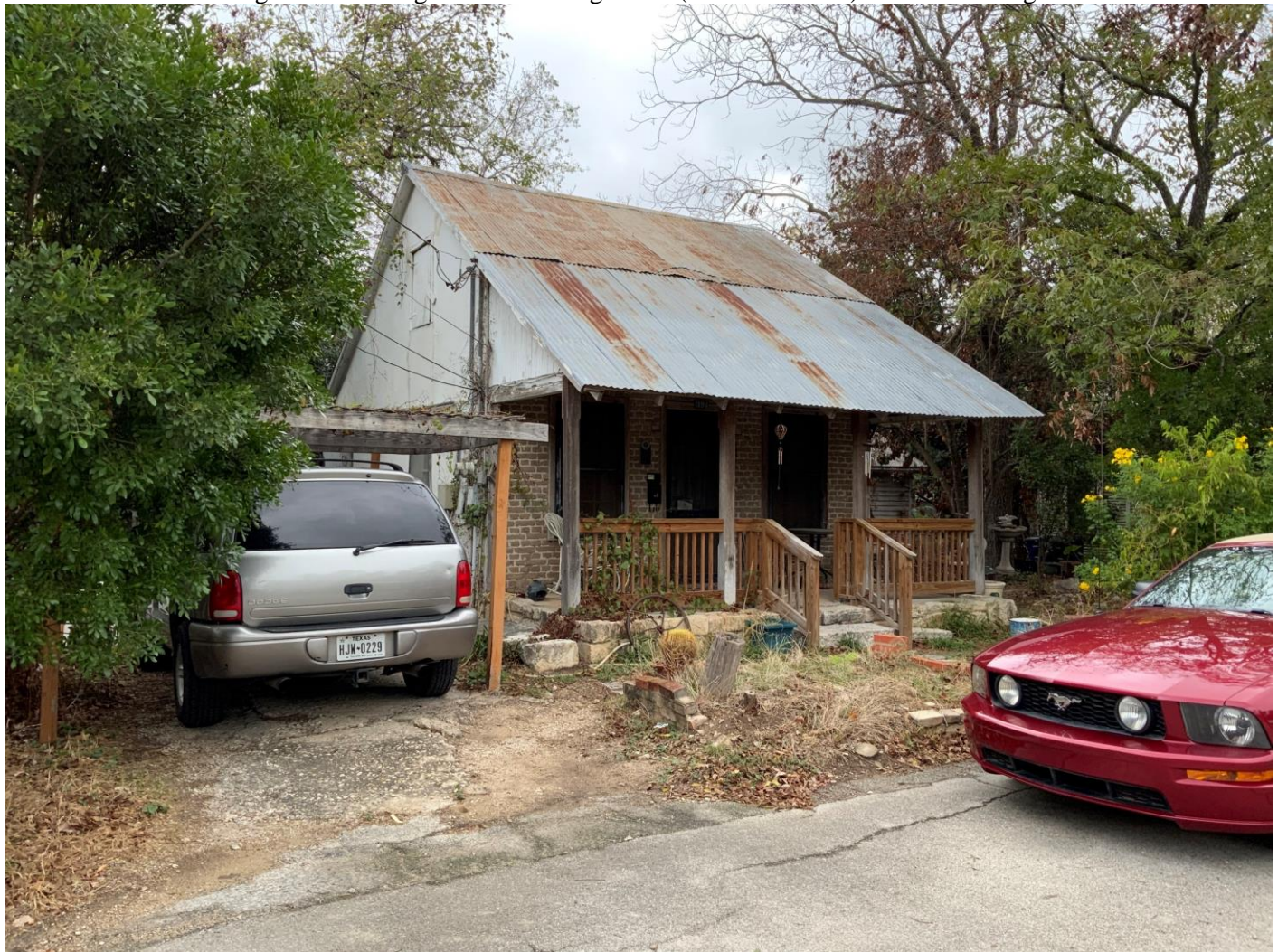
Photo 10. Camera facing north showing the contributing house (Resource 944C) at 374 W. Bridge Street.
