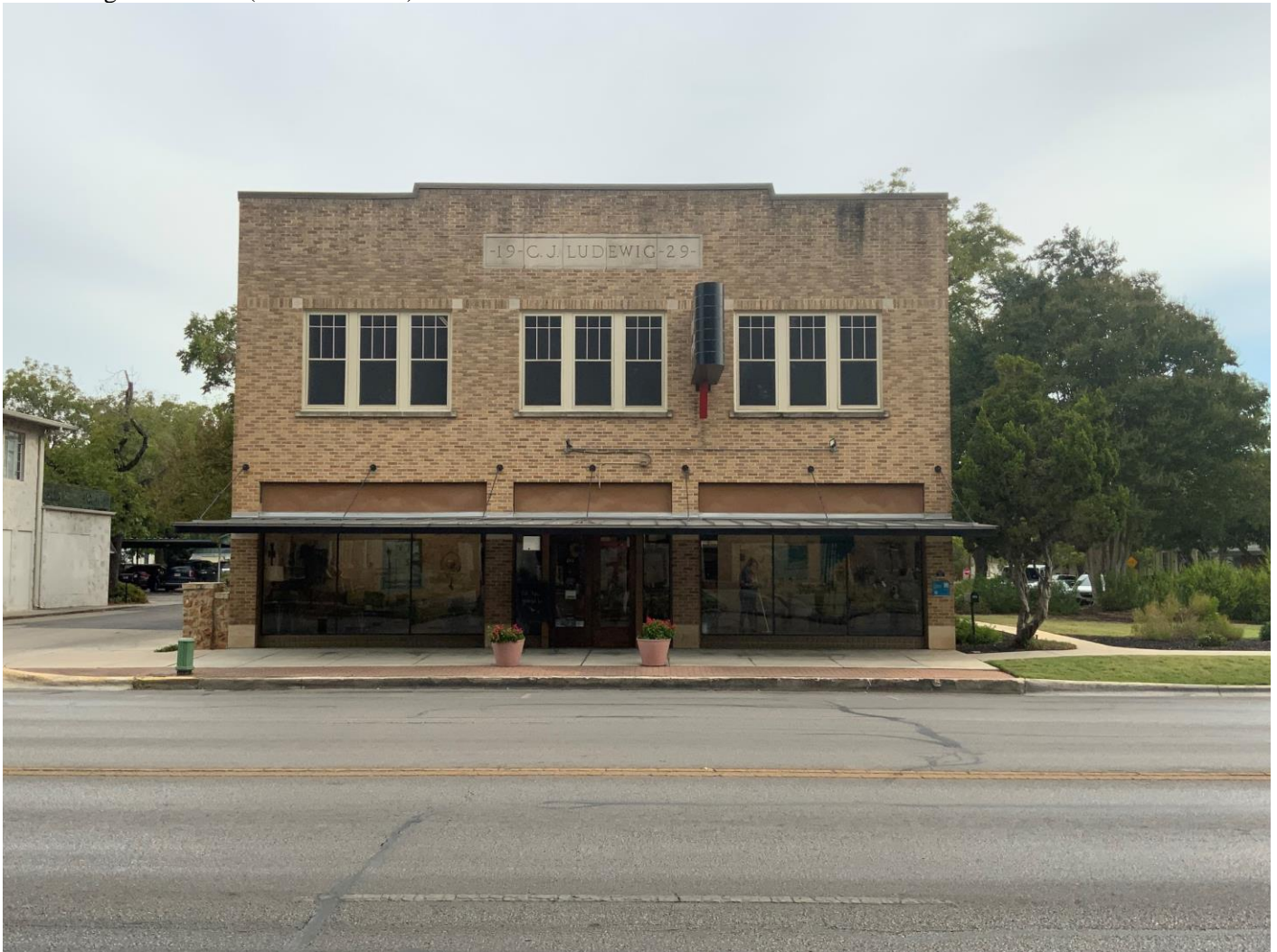
Photo 54. Camera facing northeast showing a contributing two-part commercial block Commercial style building at 283 S. Seguin Avenue (Resource 85A).
