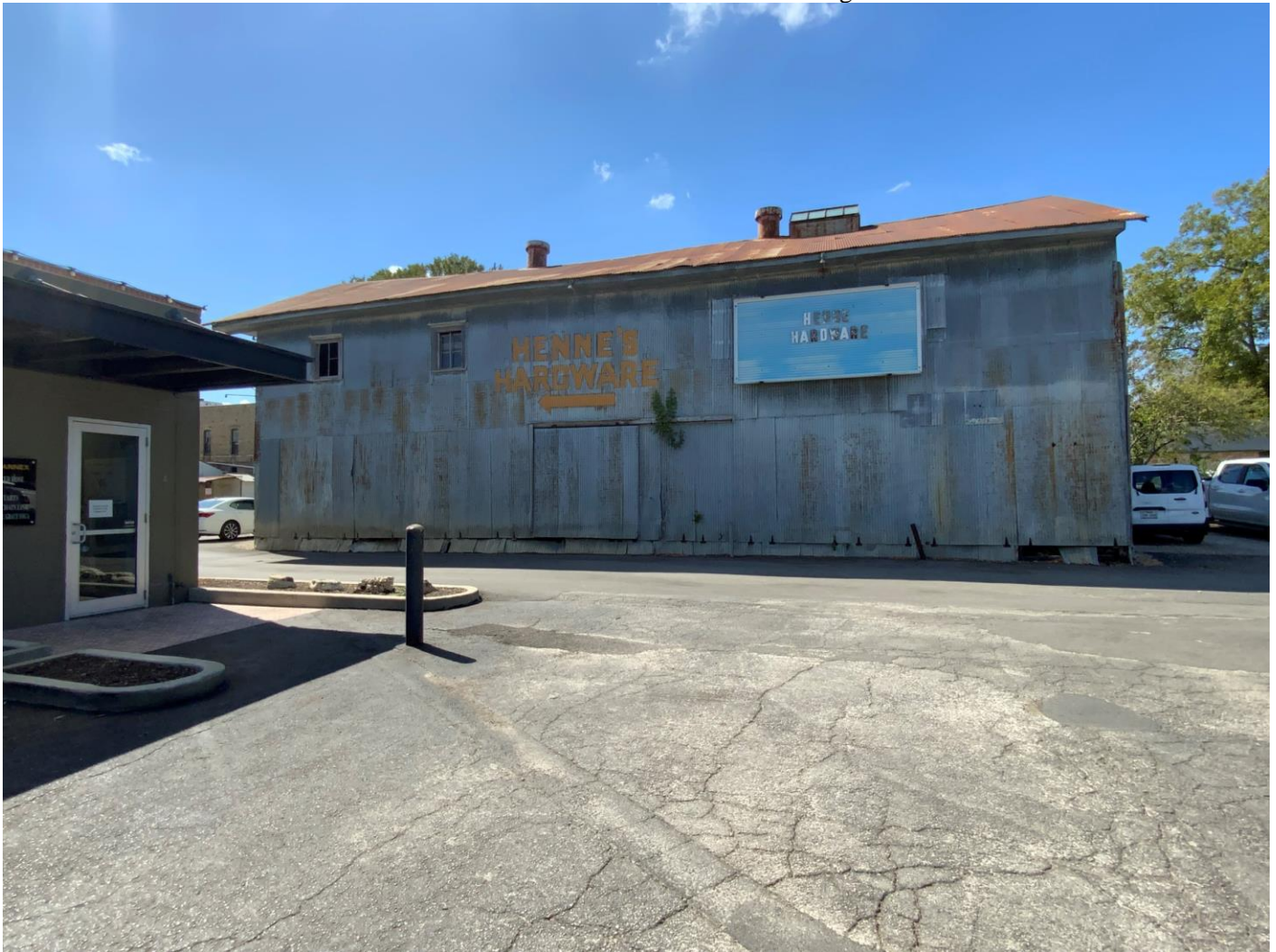
Photo 12. Camera facing south showing the contributing Henne Hardware warehouse (Resource 849) at 221 W. Mill Street. Note that it is set to the rear of the Henne Hardware commercial building on W. San Antonio Street.
