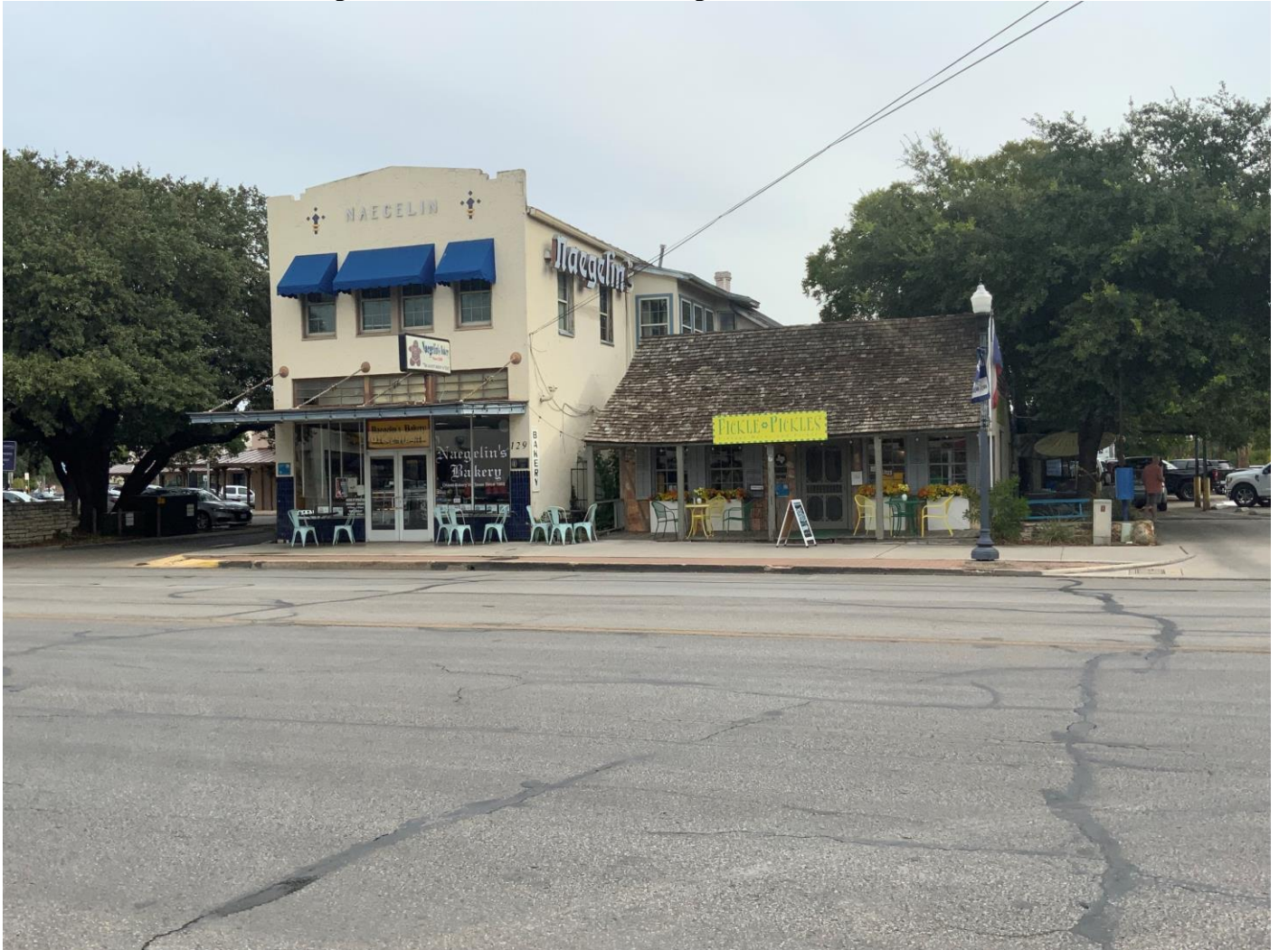
Photo 41. Camera facing north showing Naegelin's Bakery (Resource 70B) and the Stephen Klein House (Resource 70A, NRHP 1970) at 129 S. Seguin Avenue; both are contributing.
