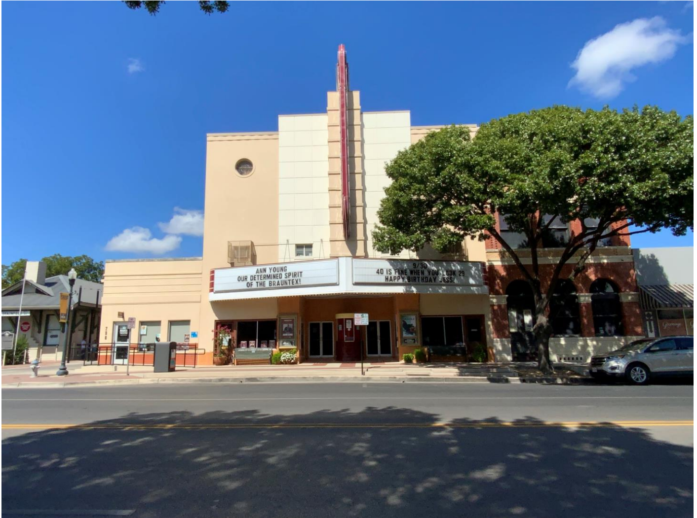
Photo 47. Camera facing northwest showing the contributing Brauntex Theatre at 290 W. San Antonio Street (Resource 837, NRHP 2008).
