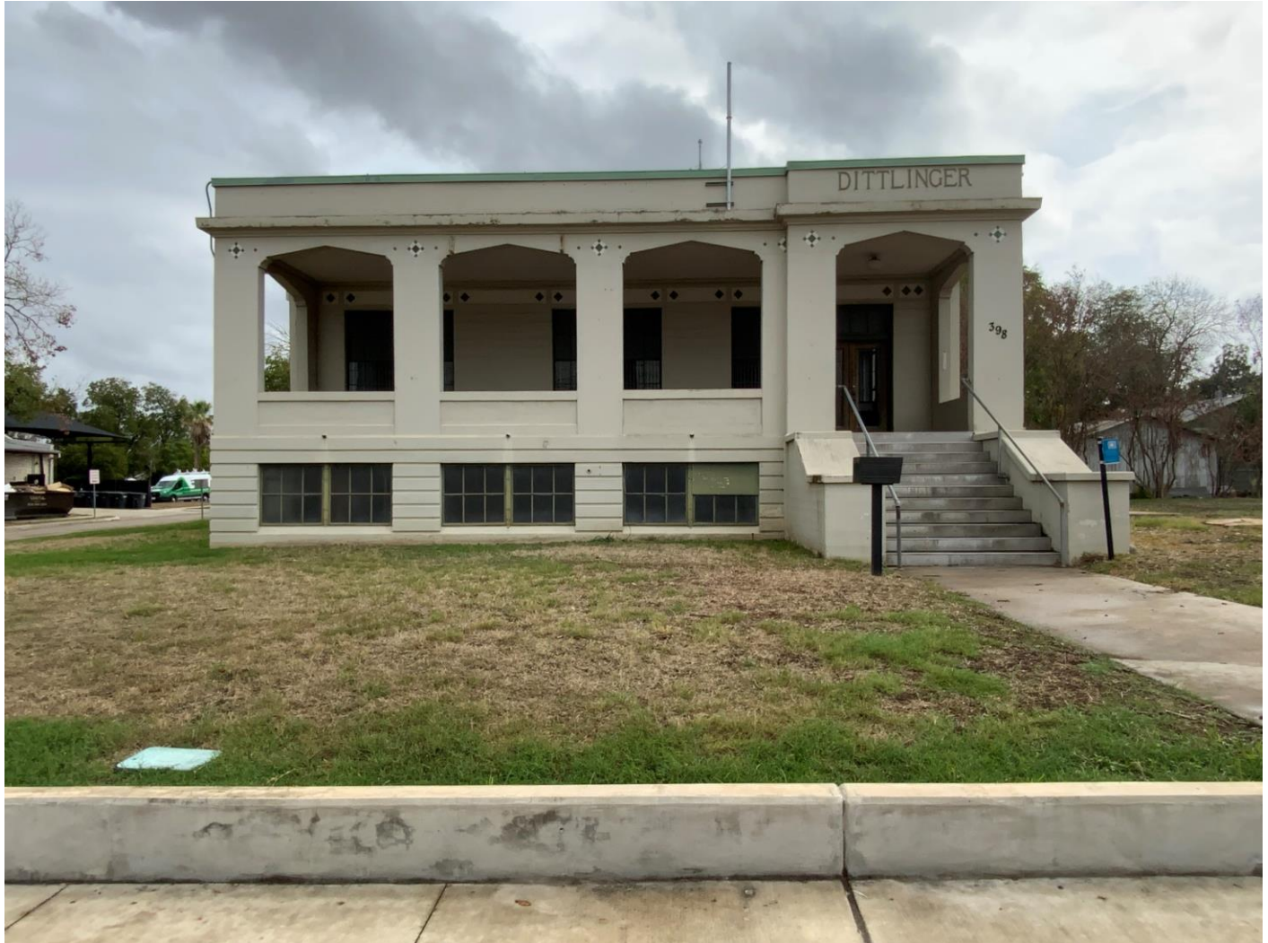
Photo 25. Camera facing southeast showing the contributing former Dittlinger office building (Resource 106) at 398 E. San Antonio Street.
