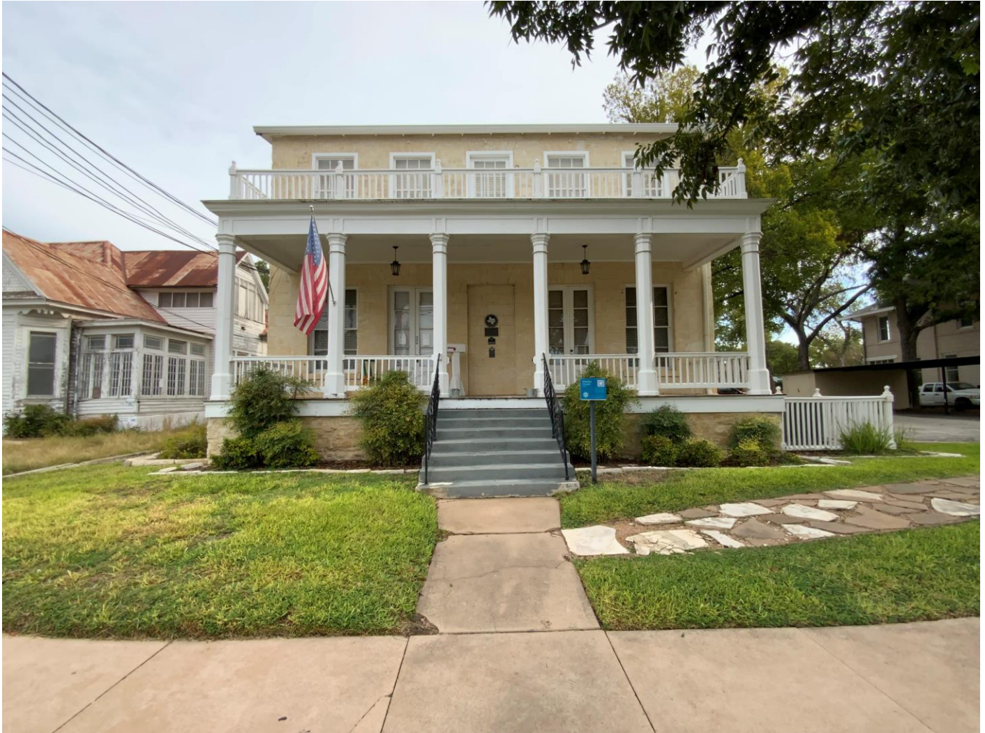
Photo 49. Camera facing northeast showing the contributing Dr. Koester House at 421 S. Seguin Avenue (Resource 222).
