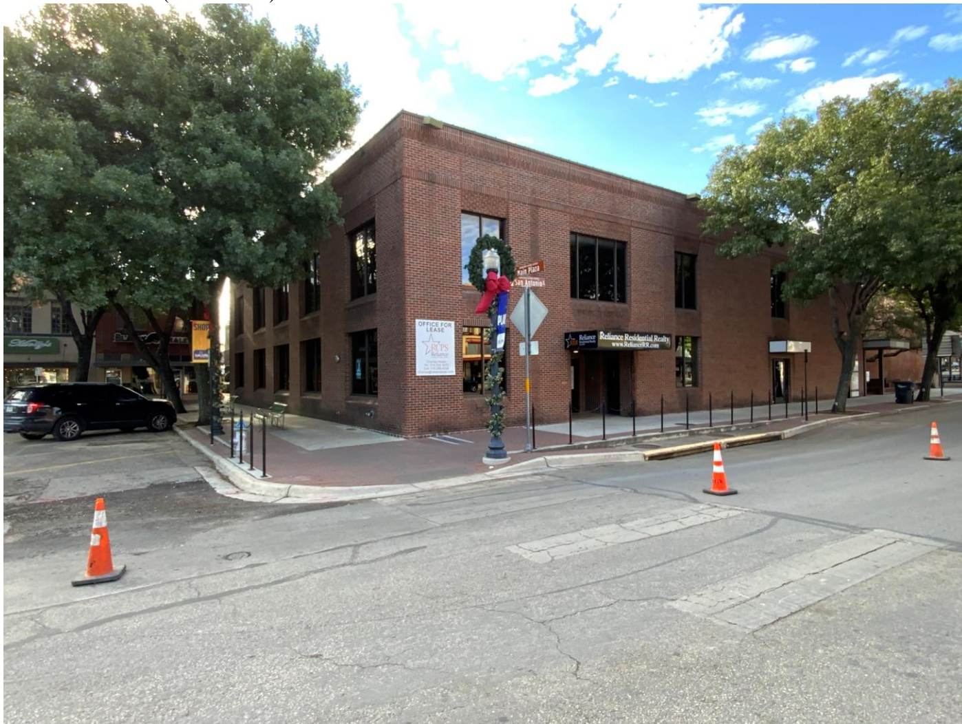
Photo 37. Camera facing south showing an altered historic-age commercial building that is noncontributing at 111 W. San Antonio Street (Resource 48).
