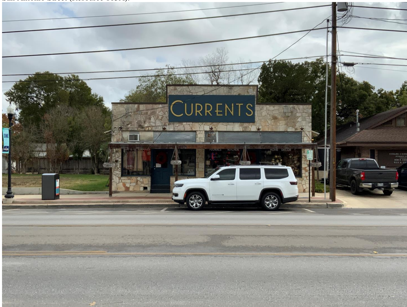
Photo 20. Camera facing southeast showing the contributing commercial building with residence at the rear at 364 E. San Antonio Street (Resource 103A).
