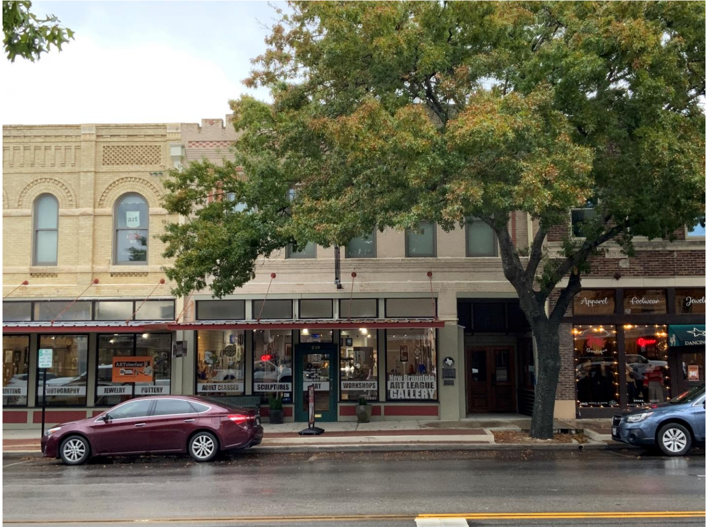
Photo 43. Camera facing southeast showing the contributing old Plumeyer Bakery (Resource 32A) at 239 W. San Antonio Street.
