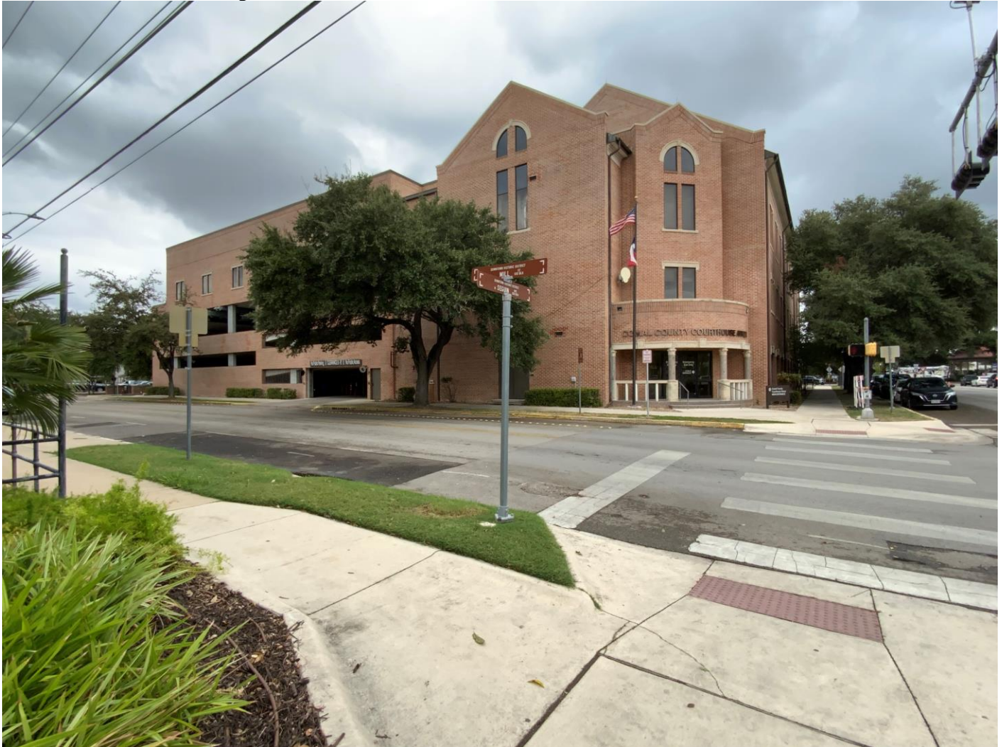
Photo 21. Camera facing southeast showing the noncontributing, non-historic-age Comal County Courthouse Annex (Resource 863) at 188 N. Seguin Avenue.
