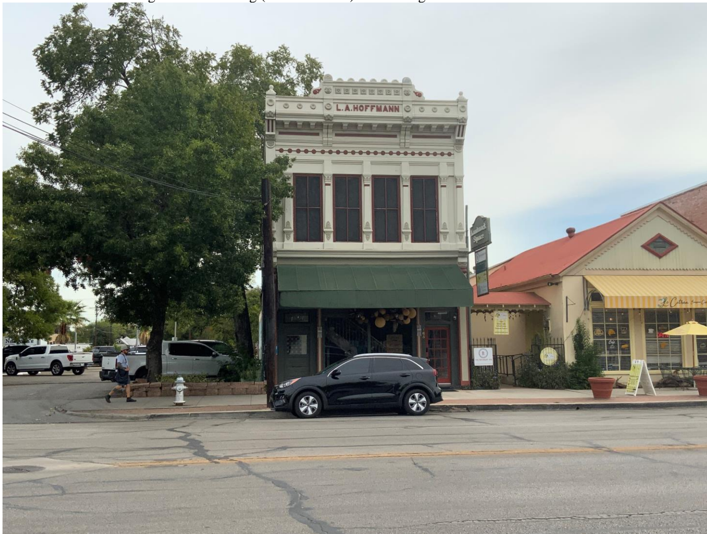
Photo 11. Camera facing northeast showing the contributing L. A. Hoffman Building (Resource 73B) at 167. S. Seguin Avenue. The contributing Krause Building (Resource 73A) is to the right.
