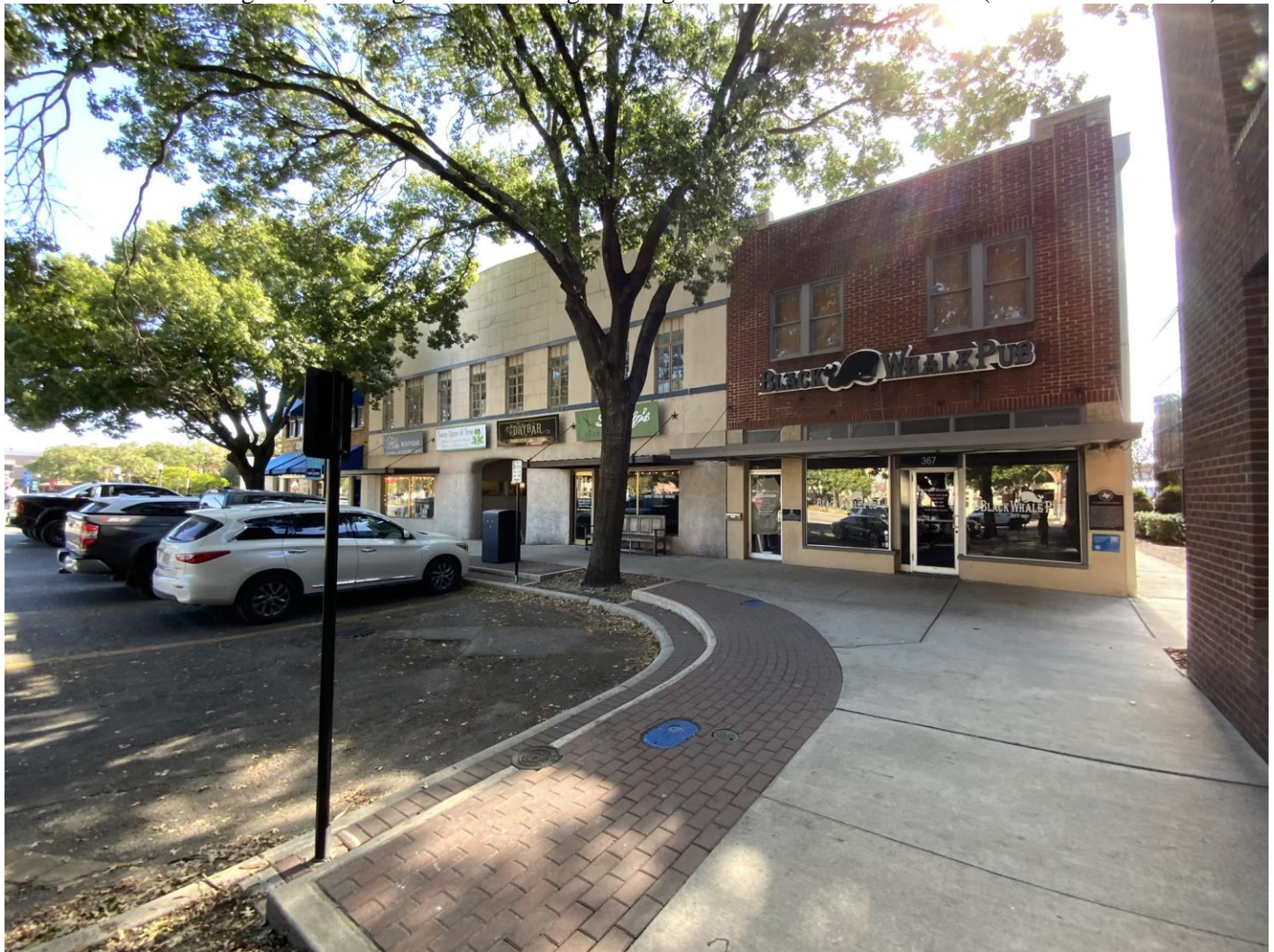
Photo 3. Camera facing east, showing the contributing buildings at 343 and 367 Main Plaza (Resources 50 and 49).
