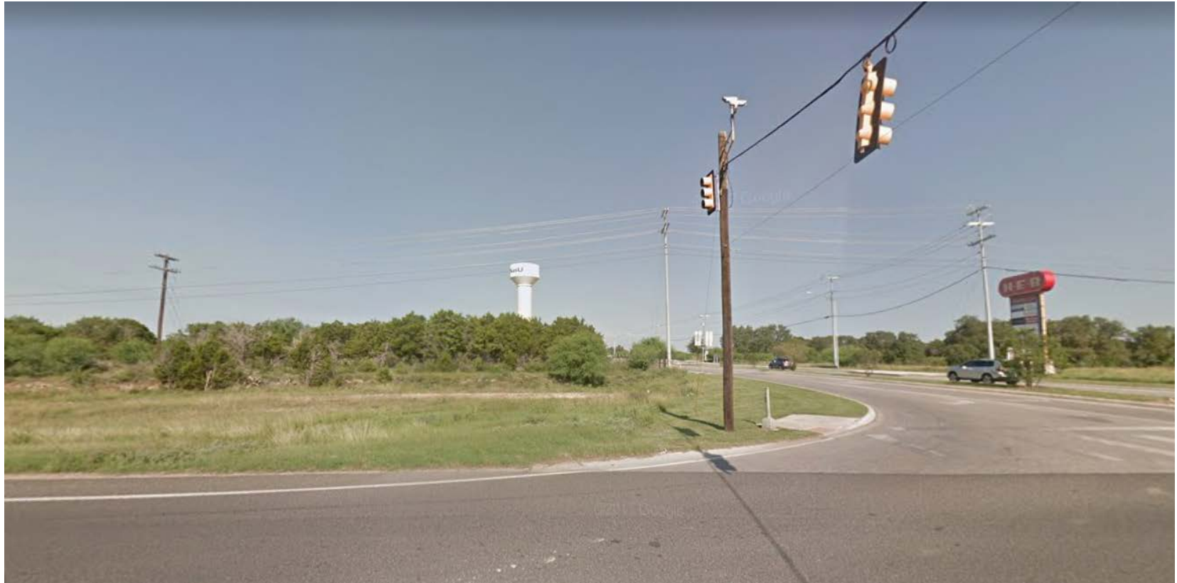
Subject property at the intersection of Loop 337 and Oak Run Parkway
