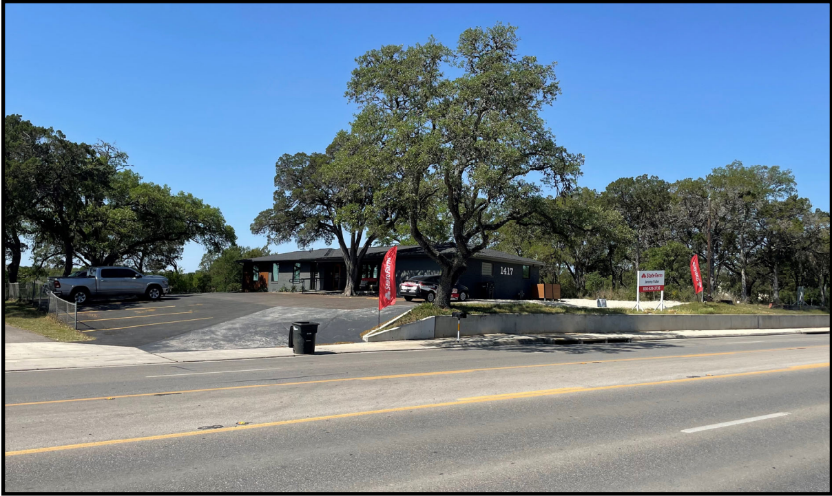
Subject Property Frontage Along N Walnut Ave Facing Southwest
