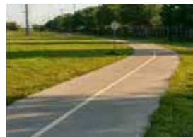
Example: Utility Corridor Trail
