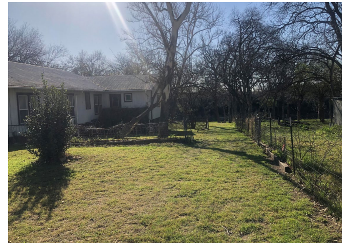
5e - View of subject property from the SW corner at Granada
