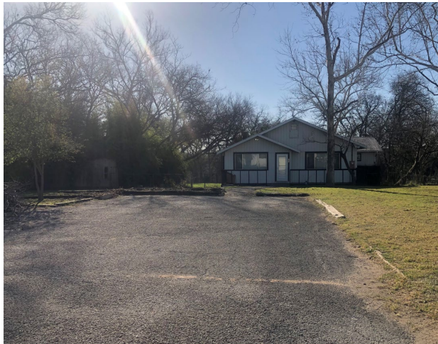
5d - View of subject at drive way entrance from Granada
