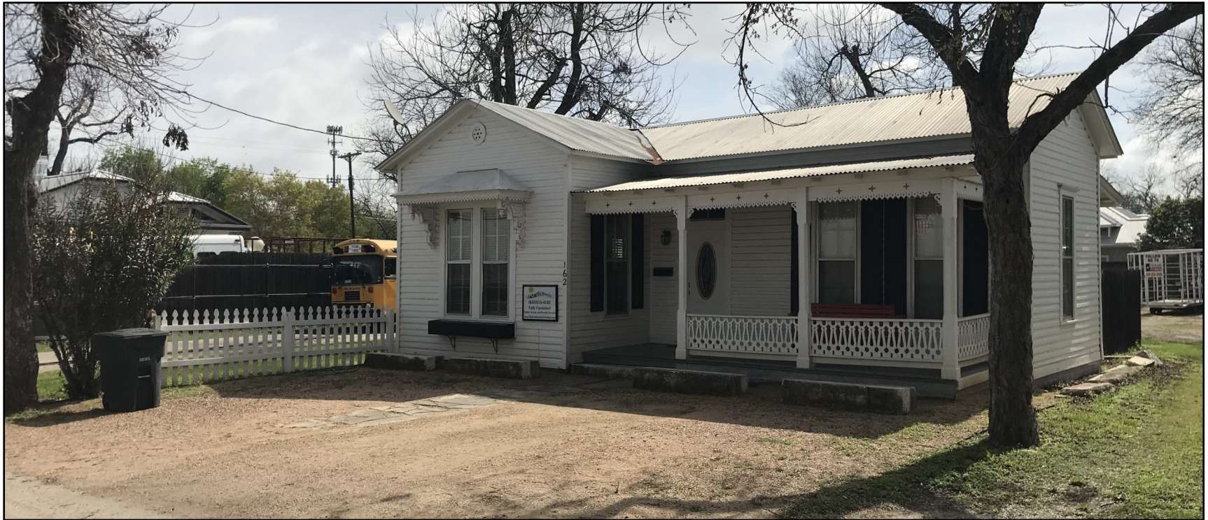
Subject property from Meusebach Street.
