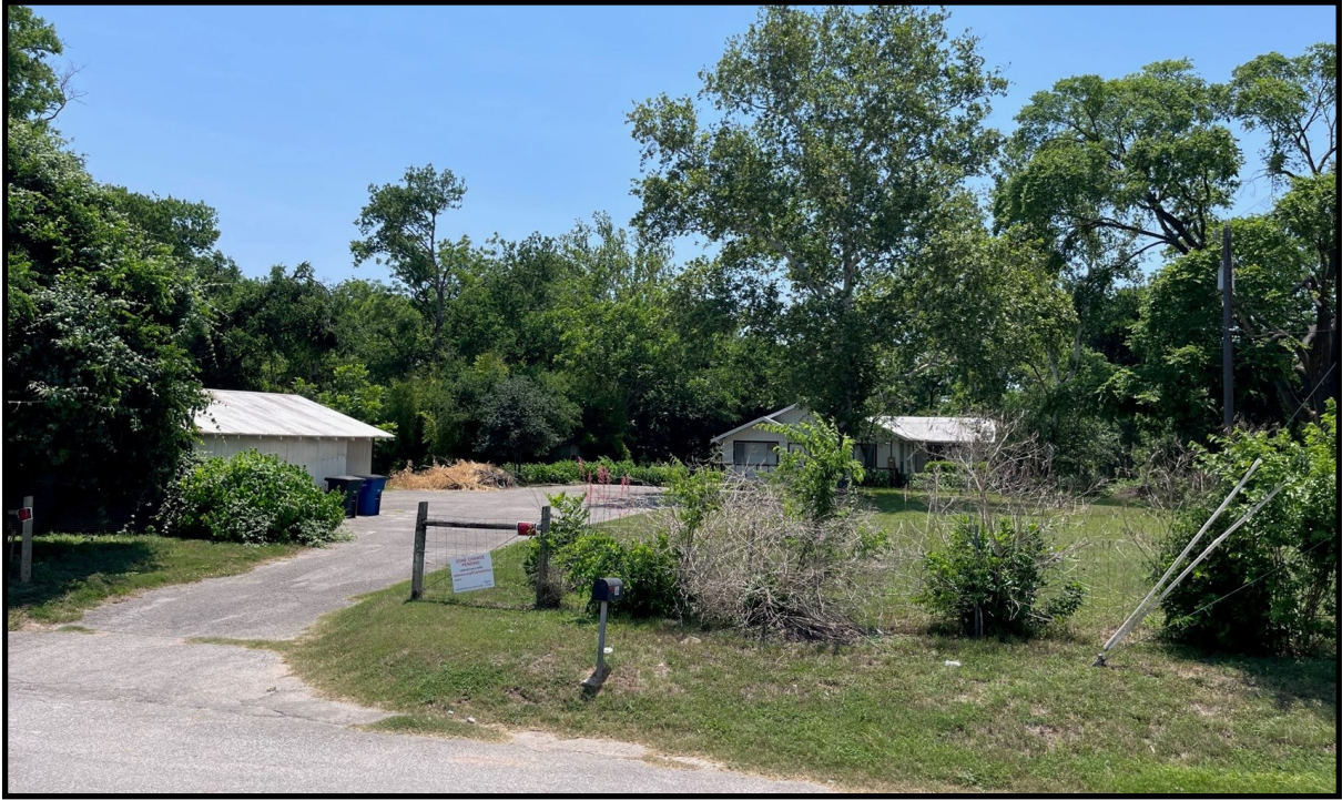
586 Granada Drive property frontage
