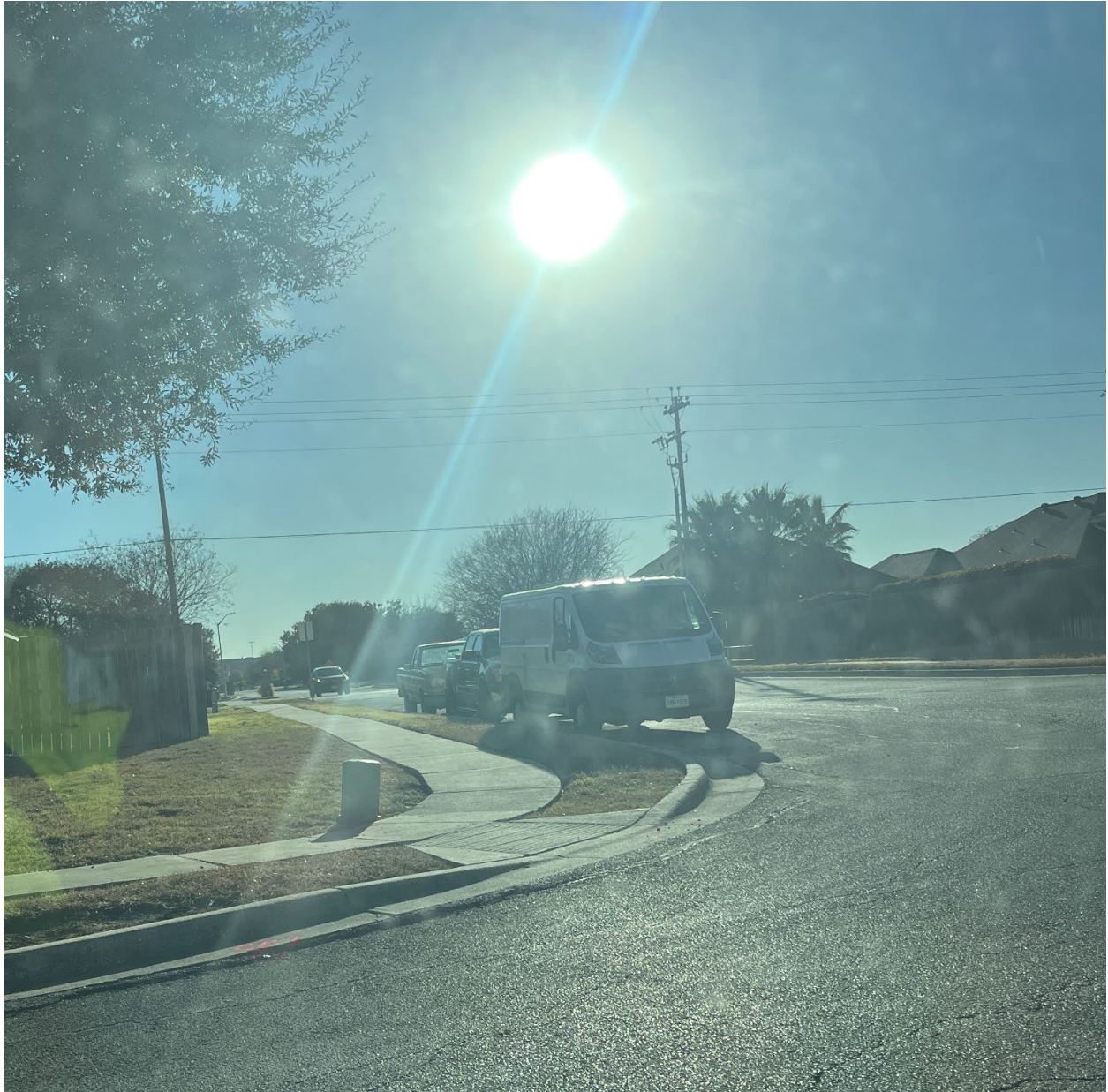
Figure 2 – ADA ramp and pavement before the 2023 Bond Citywide Street Improvements project.
