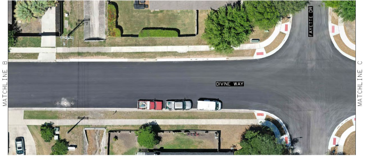
Figure 3 – Current, improved pavement and ADA ramps at the subject intersection following the 2023 Bond Citywide Street Improvements project.
