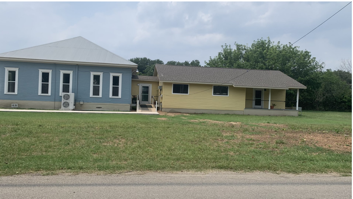
511 E North St—View from E North St
