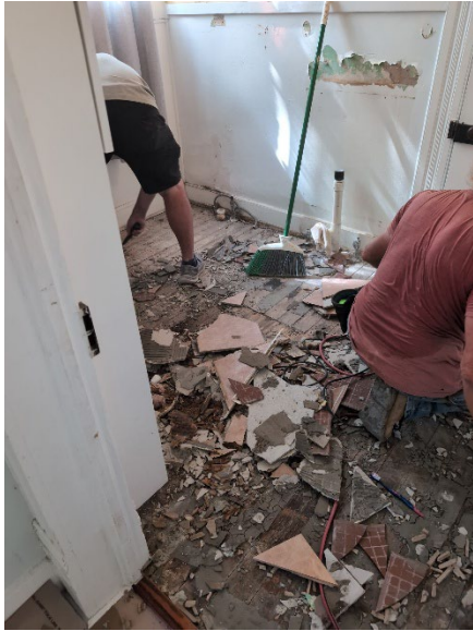
Original Bath Room
