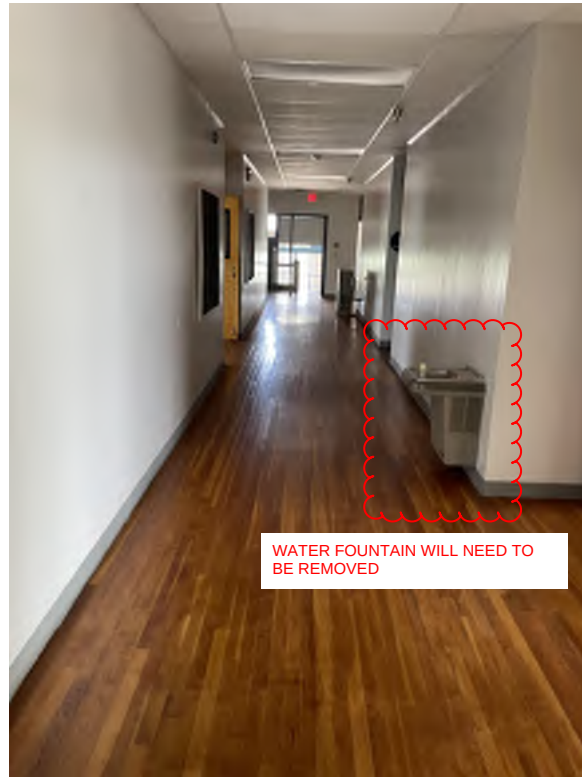
Figure 25: Third Floor Level Corridor
