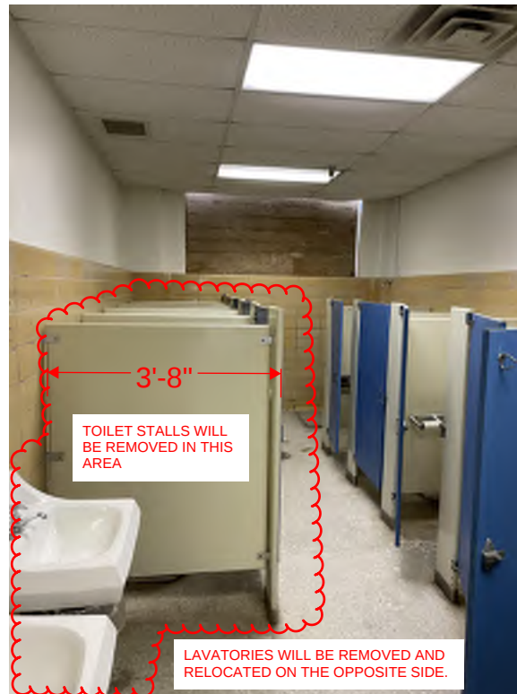
Figure 15: First Floor Basement Girls Restroom
