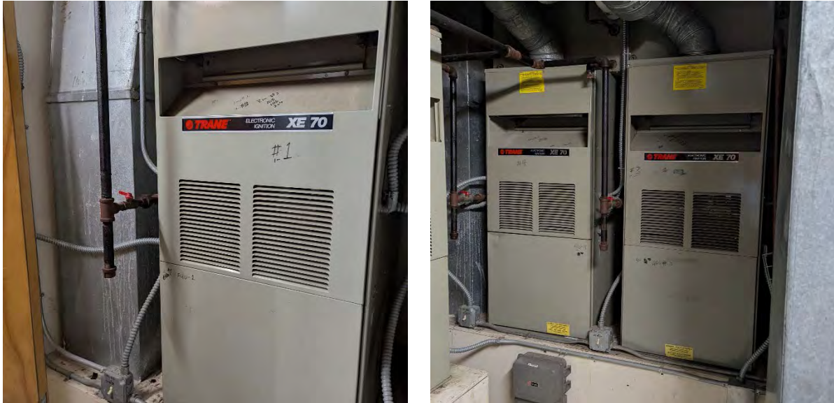
Figure 7. First floor vertical air handlers
