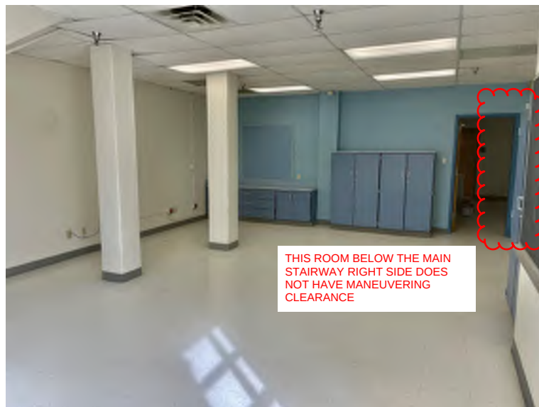
Figure 12: First Floor Basement interior doors
