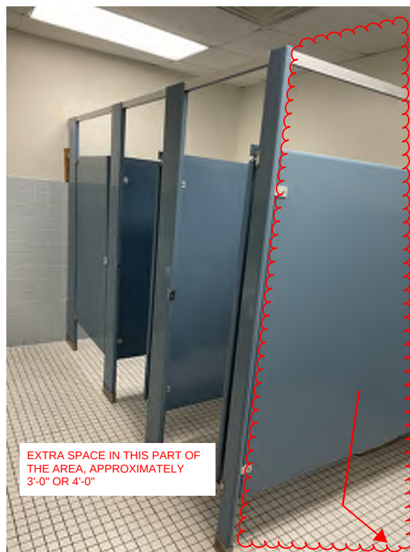
Figure 28: Third Floor Level Women's Restroom
