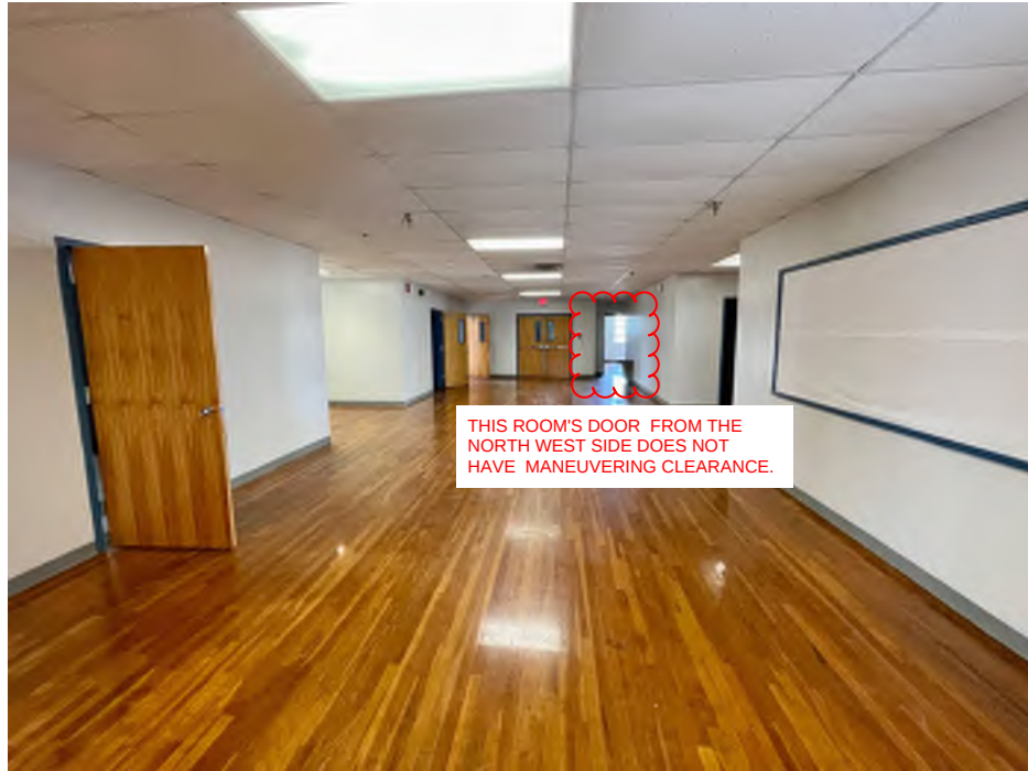
Figure 21: Second Floor Main Level Lobby
