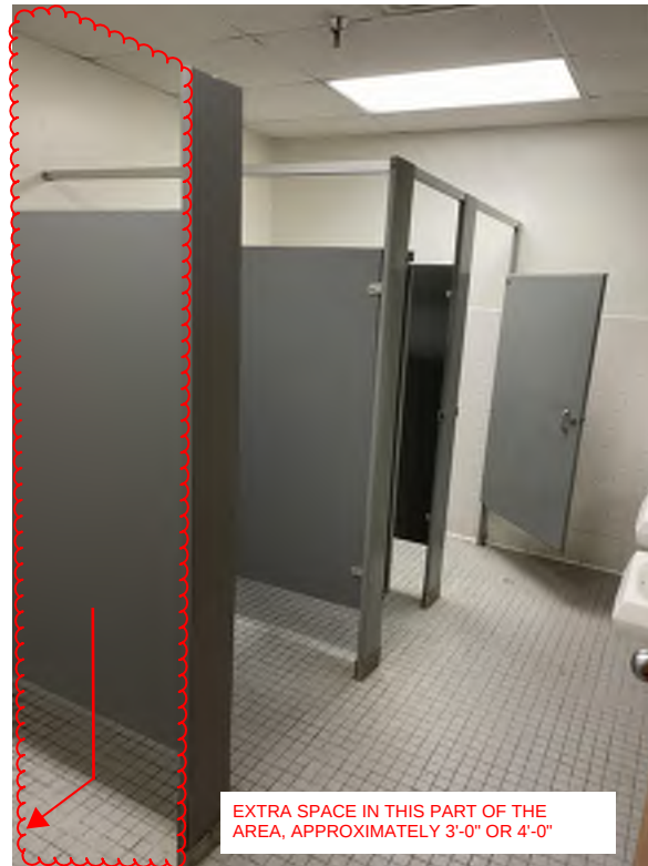
Figure 27: Third Floor Level Men's Restroom
