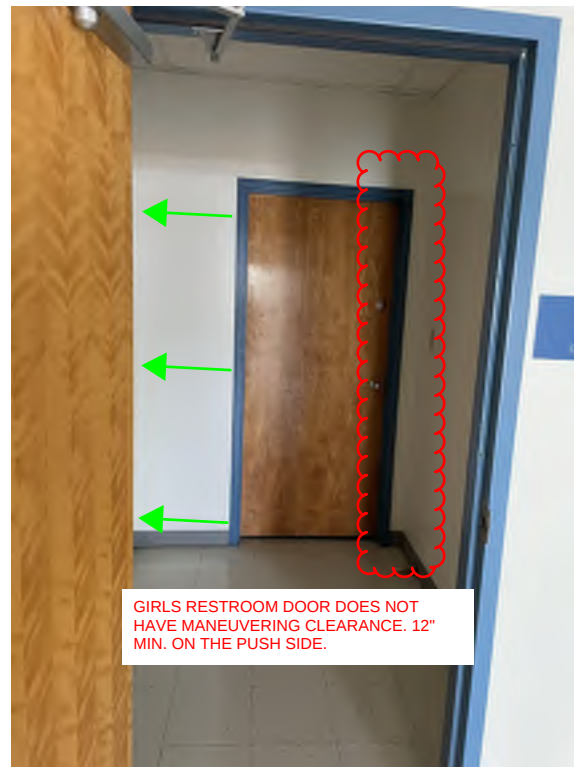
Figure 14: First Floor Basement Girls Restroom
