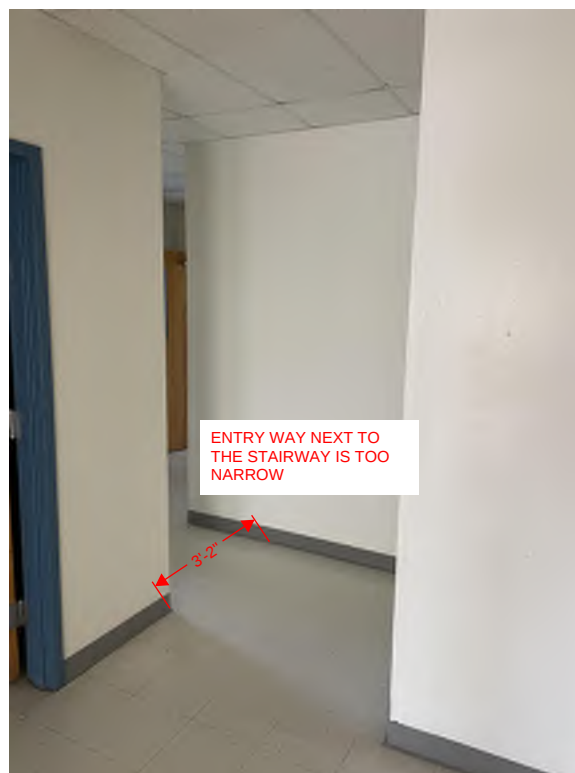
Figure 18: First Floor Basement Stairway
