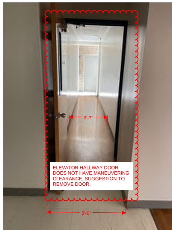
Figure 10: First Floor Basement Elevator Hallway
