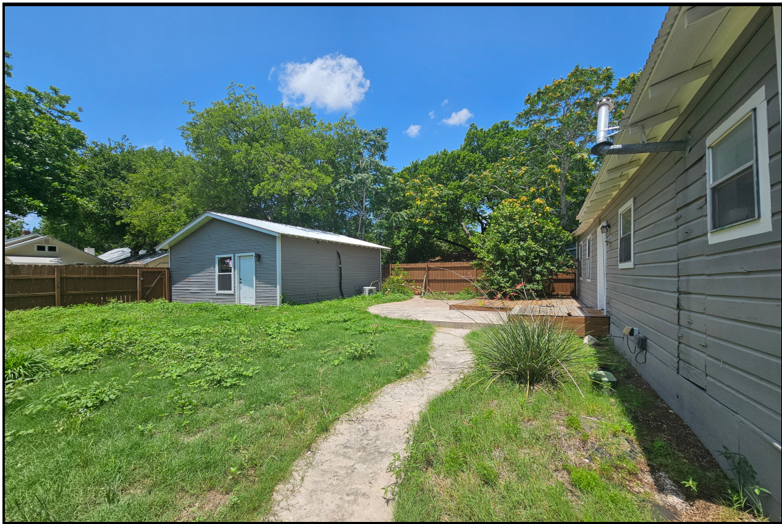
574 S. Academy Ave. Rear of Property
