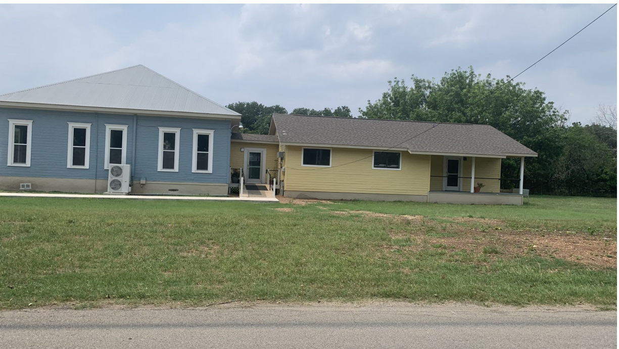
511 E North St—View from E North St
