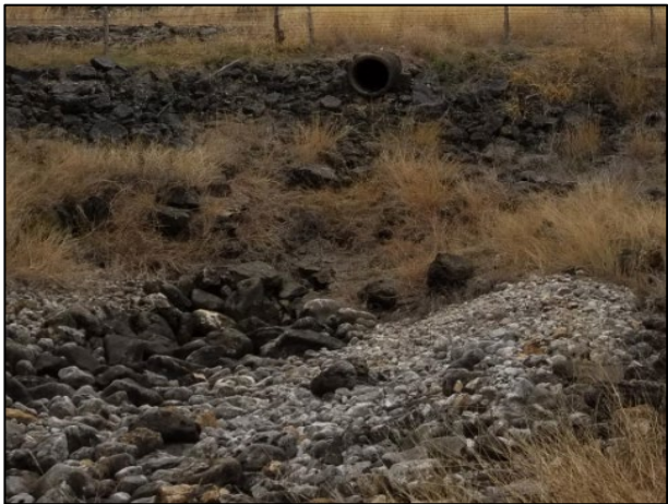
Outlet Pipe and Plunge Pool (2020)
