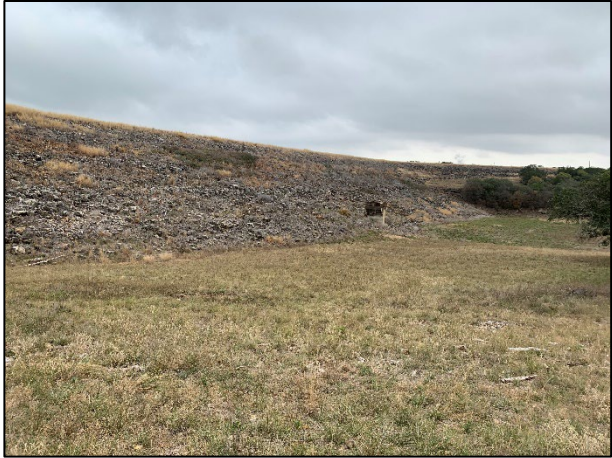
Upstream Embankment Showing Rock Blanket (2020)
