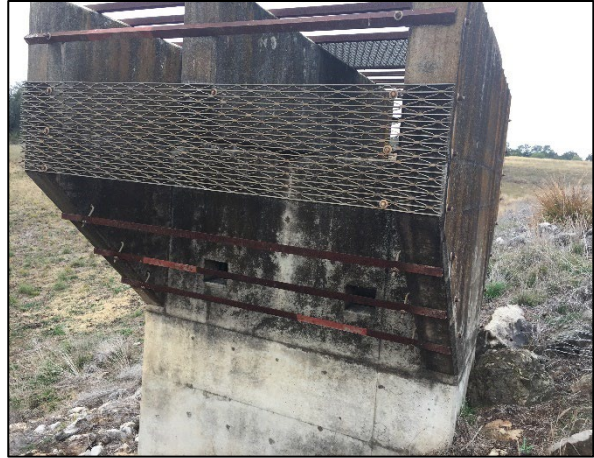
Inlet Structure with Low Level Ports (2020)
