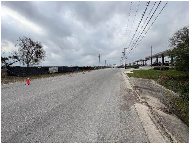
Looking west along West San Antonio Street, subject on the right
