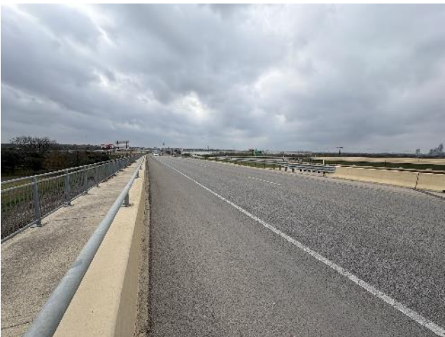
Looking south along Loop 337, subject on the left
