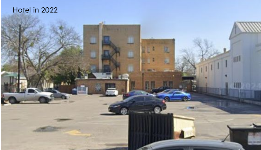
Current, under construction
