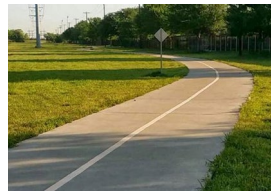
Example: Utility Corridor Trail
