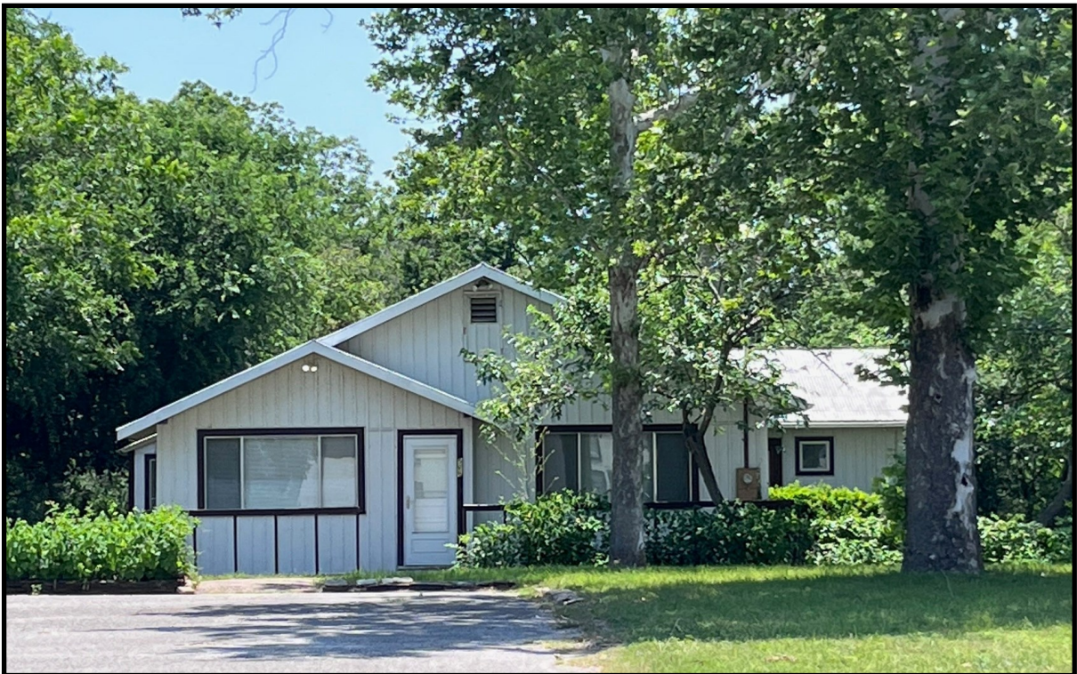
586 Granada Drive residence
