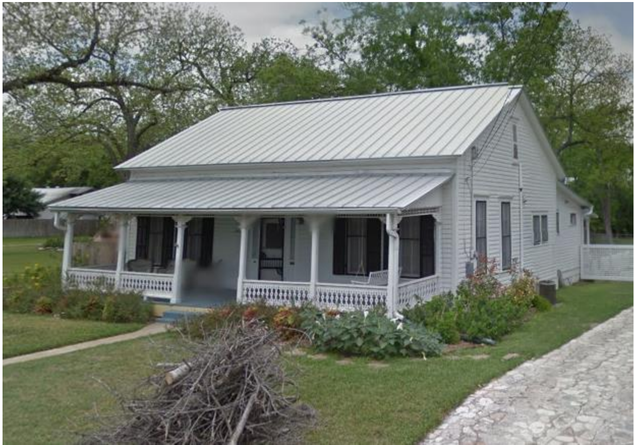
586 W. Mill Street, after rehabilitation
