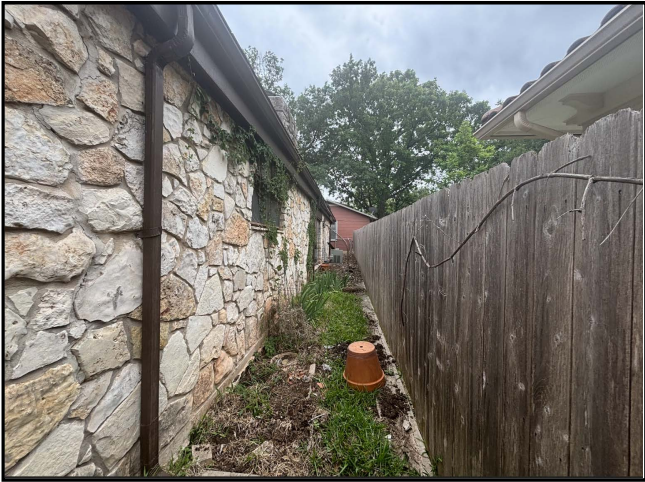
Rear of house
