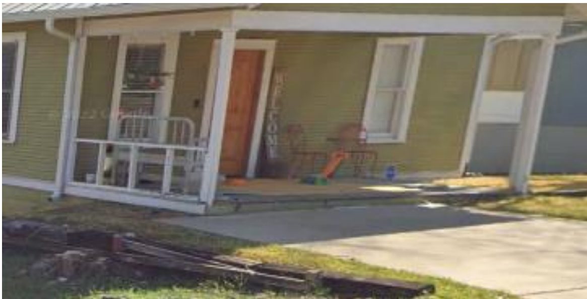
Note: The rot completely rotted out this left side rail to which it had broken off near the post.
