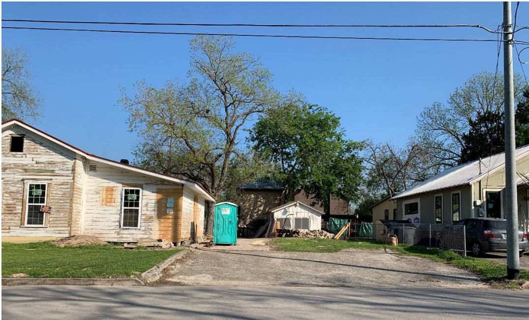
Parking area being improved
