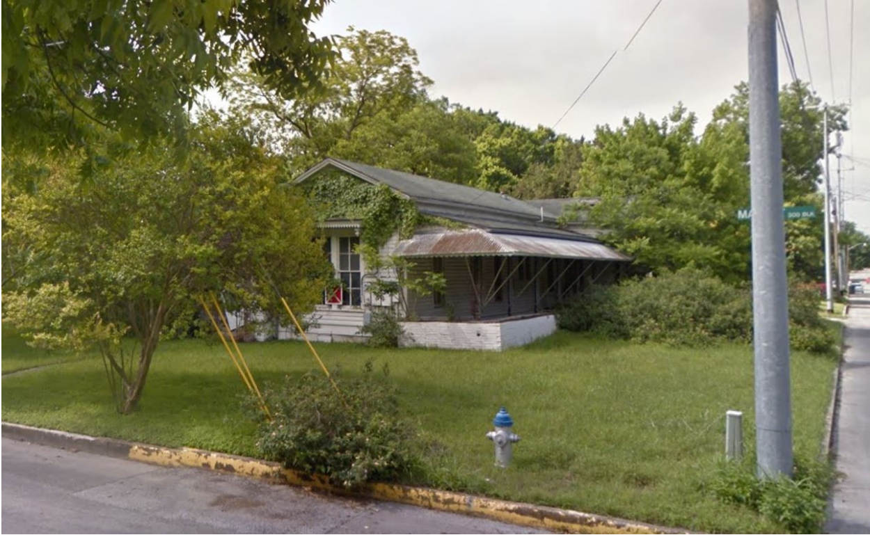
Subject property before renovations began
