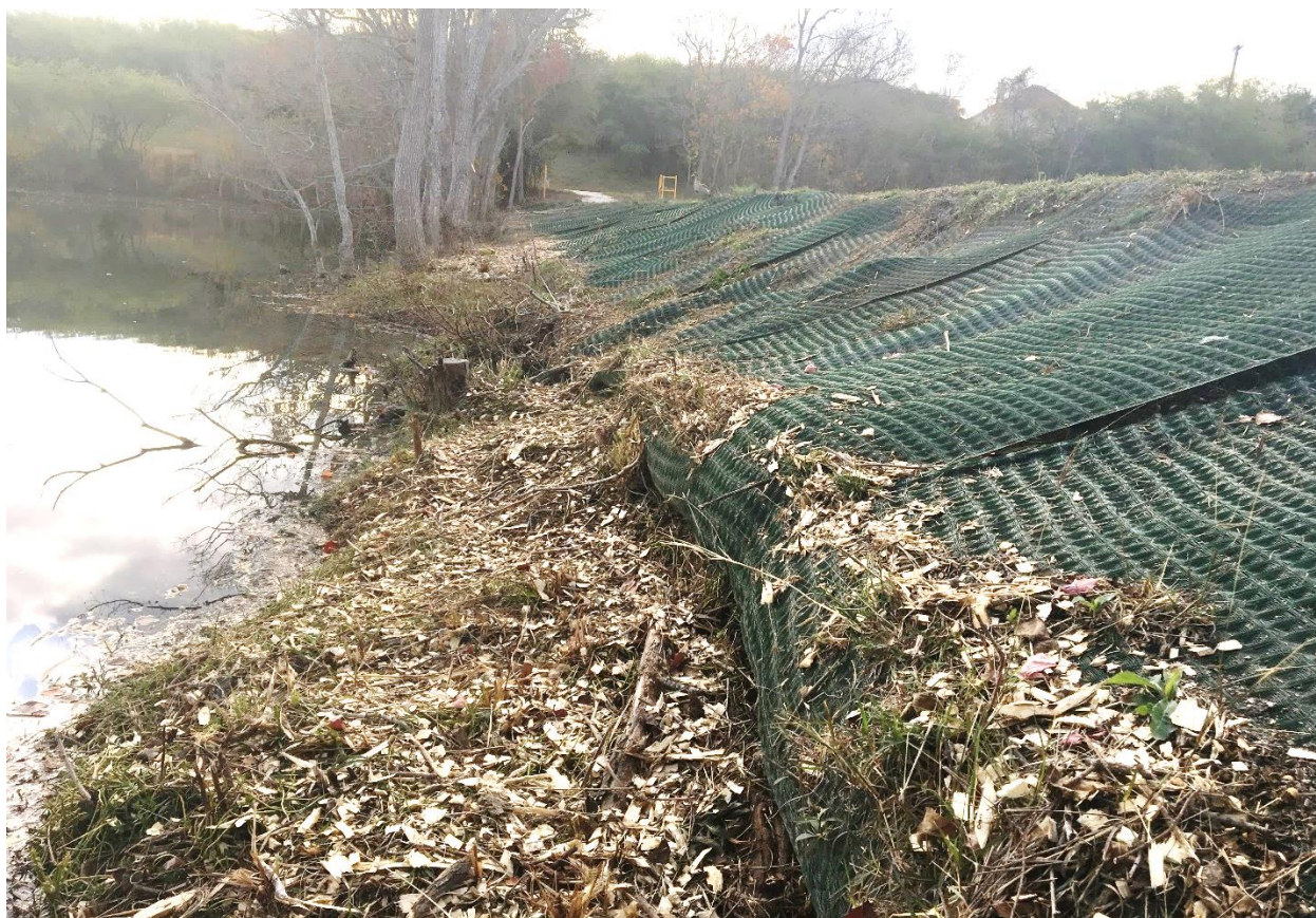
Photo 6: Erosion at Downstream Toe of Spillway
