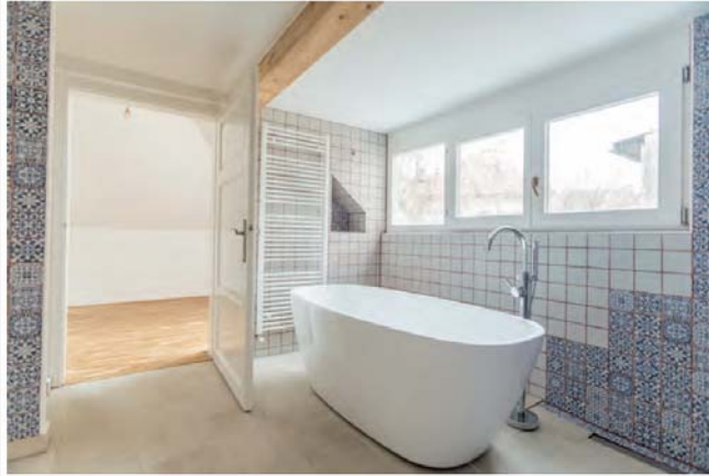
An overflow is not required for a bathtub
