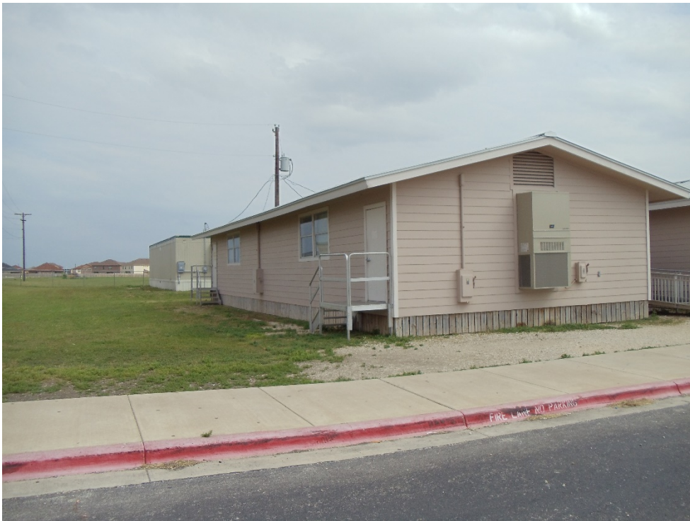
The subject modular buildings currently located at Canyon Middle School
