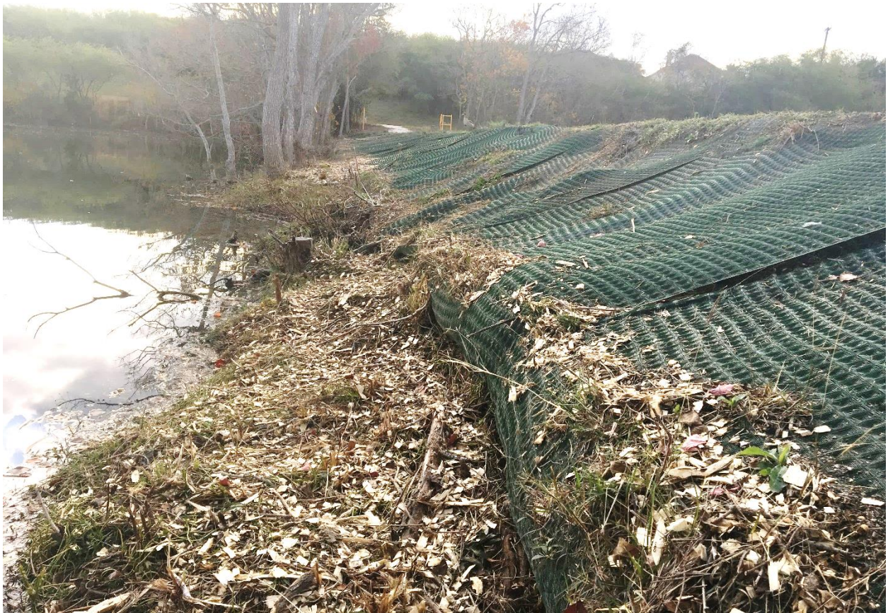
Photo 6: Erosion at Downstream Toe of Spillway
