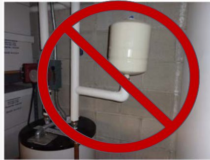
Unsupported thermal expansion tank
