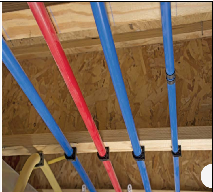
Air testing of PEX water piping is permitted
