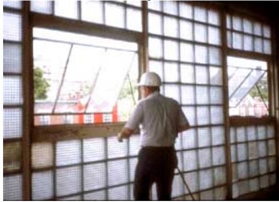
Preparing historic steel windows for repairs and re-finishing.
