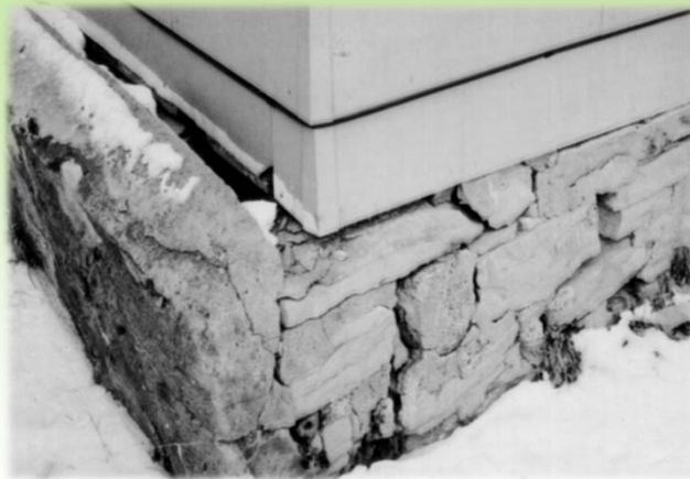
Major Damage to a Foundation Wall
