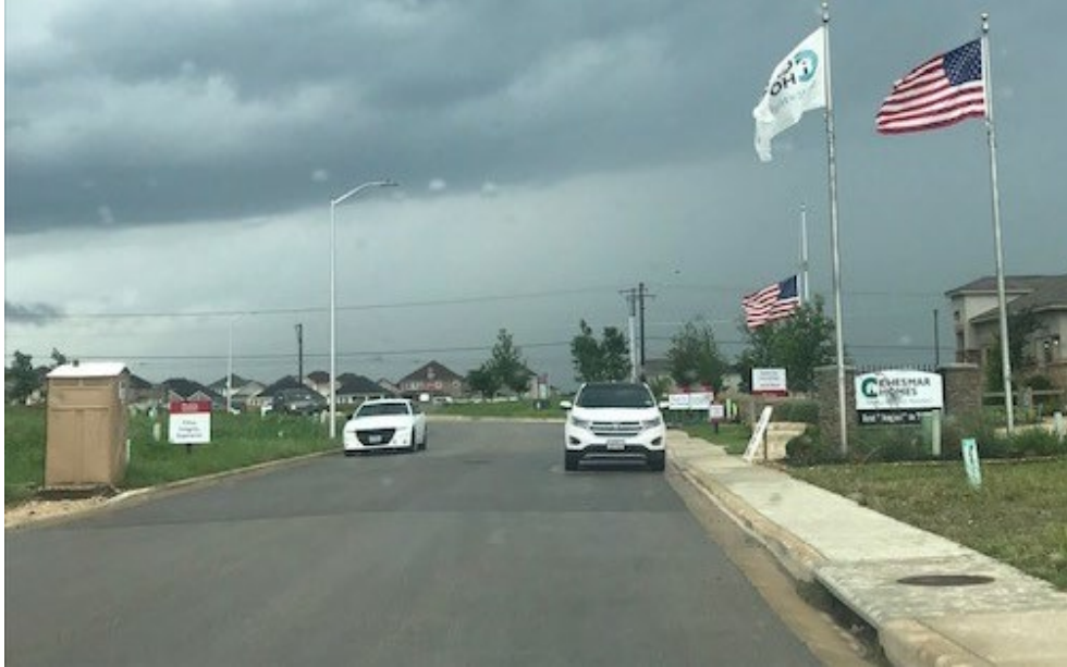
Cars parked on either side of Willowbrook in front of the model home (721 Willowbrook). Road is wide enough for a third vehicle to drive through between them.
