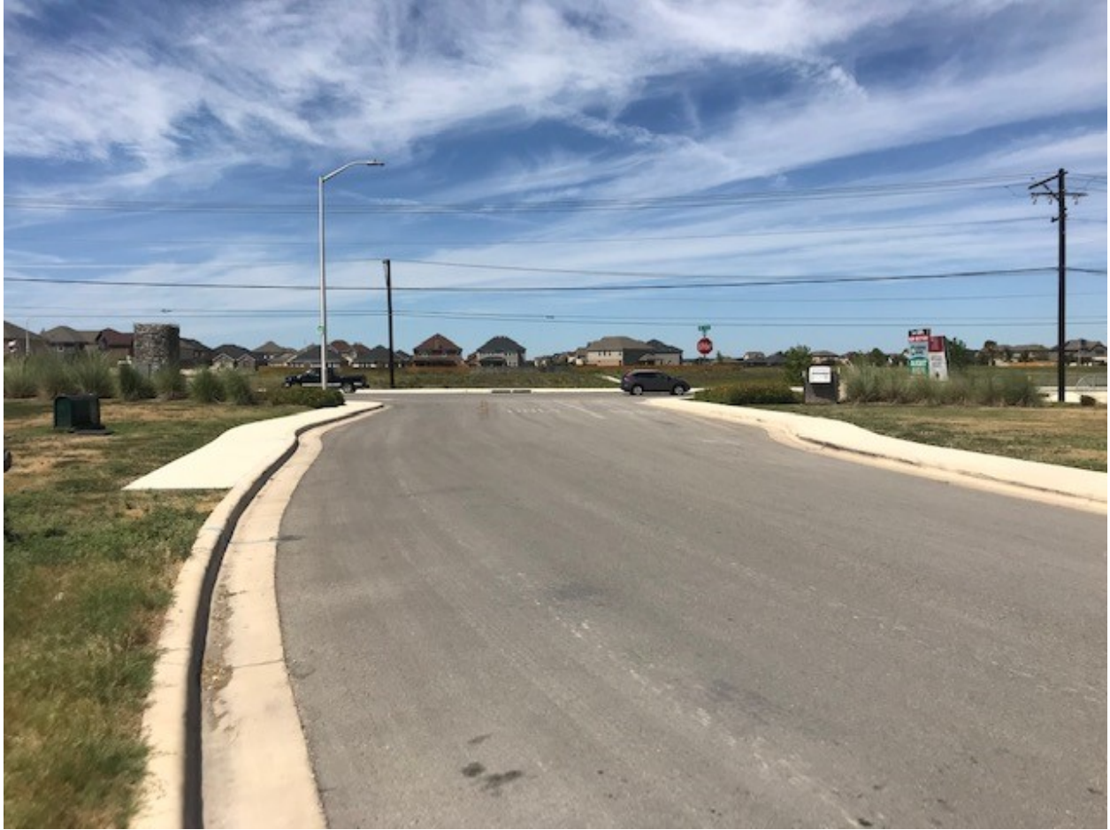
Pavement width measured at 36 feet at entrance of subdivision where road is striped for 3 lanes. Pavement width further within subdivision measured at 30 feet.
