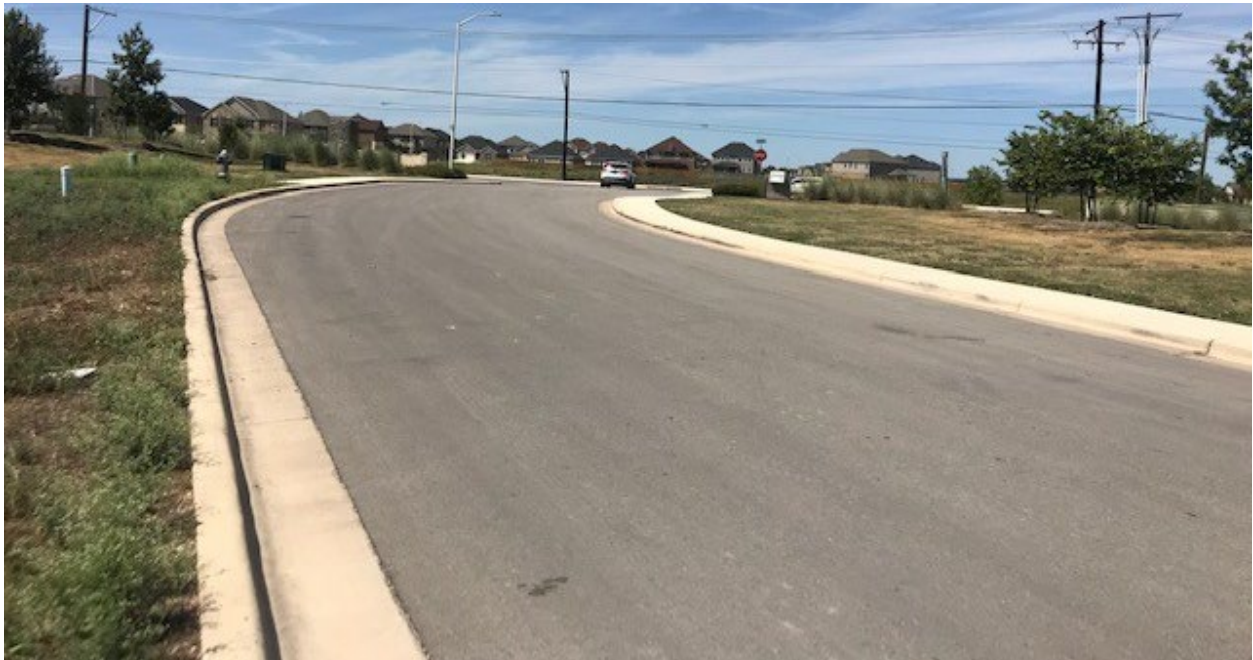
Visual of roadway width and current state of sidewalk at front of subdivision. Gap is visible on the southeast side of Willowbrook.
